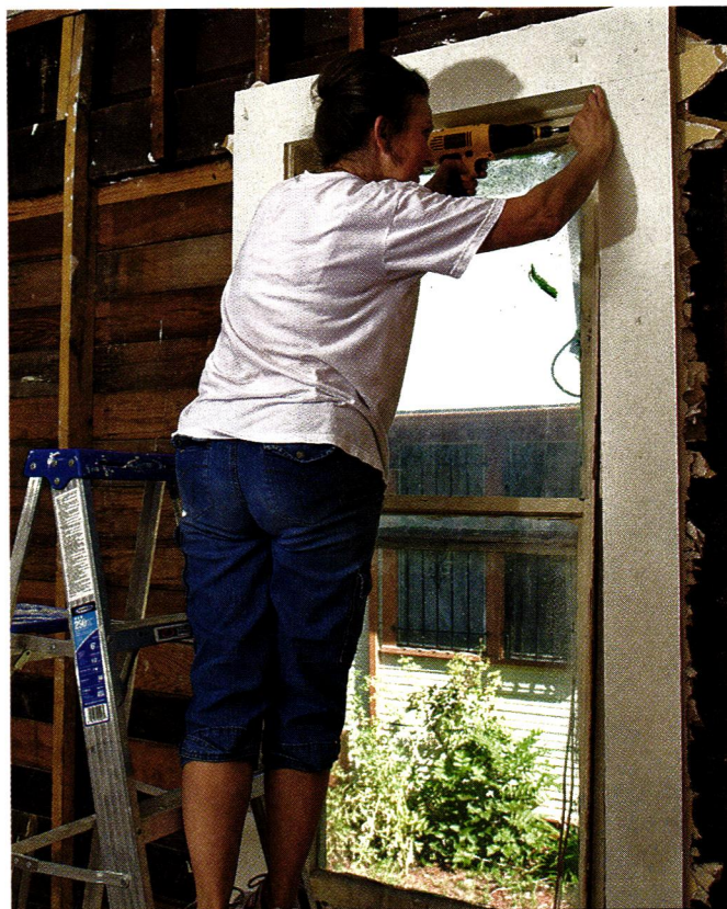
Pam begins the window restoration by removing nails and screws and carefully prying off trim and interior stops.
