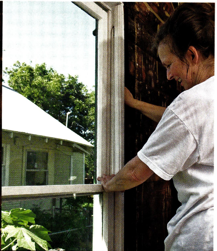
Once both sashes are in place, Pam checks the rope again and adjusts as necessary before replacing the interior stops and trim.
