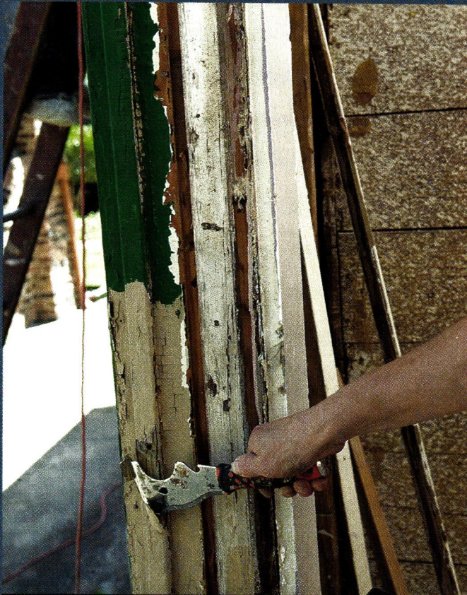
Armed with her 5-in-1 painter's tool, Pam begins cleaning up the window frame by scraping away layers of flaking paint.
