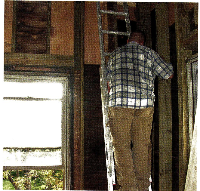
Installing new framing and sistering beams were critical to shoring up the tower.
