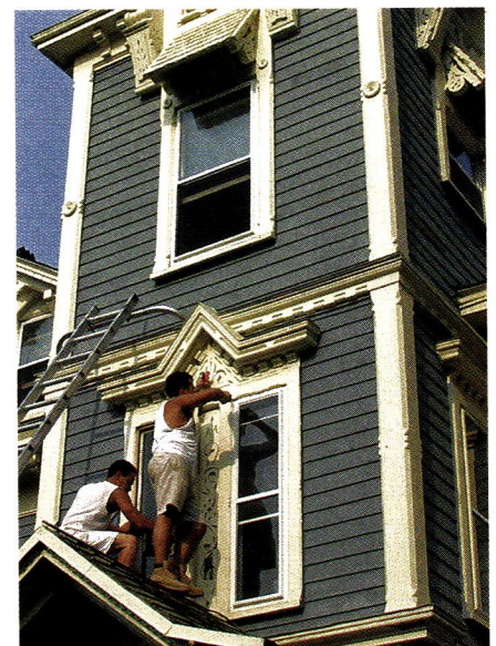
Craftsmen stripped and painted exterior decorative elements, and restored windows.
