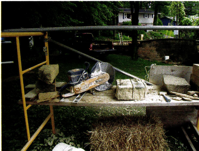
Cut the new stone to size (here, using a Partner saw). Remember to leave enough depth to work the surface to the desired texture.
