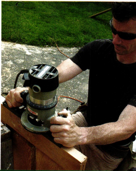
After marking the new location of the hinges, Mark uses a router and mortising jig to cut the mortises. For mortises on the jamb leg, he takes a chisel to the corners to make them nice and square. Next, he assembles the jamb, pinning it together with just a few screws so that it's ready to be moved into position, but can still be disassembled if adjustments are necessary.
