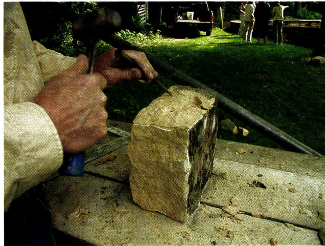
Clean up any high points along the sides of the new stone with a point chisel.
