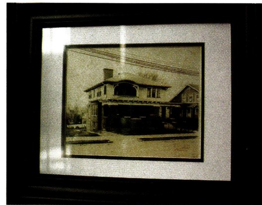
TOP: Faith's grandmother's wicker loveseat graces the upstairs sleeping porch, restored to its original use. BOTTOM: A copy of Billie McKinney's black-and-white photo of the home, which inspired the sleeping porch discovery, now hangs proudly on a wall in the living room.
