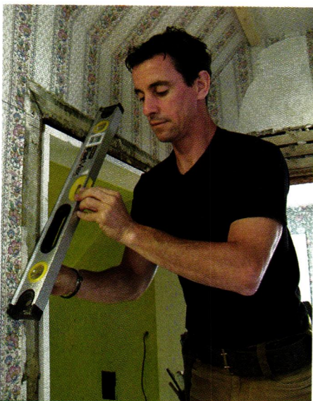
With the door jamb sitting in its new location, Mark uses a 2' level to register the assembly flush with the wall surface, then pops a nail into the top, middle, and bottom. After aligning the hinge barrels and sliding them together, Marks shims the jamb straight. Last step: Mark places a 3" deck screw through the hinge leaf and snugs it into solid framing.
