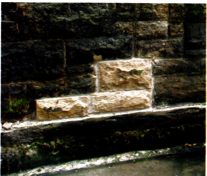
FROM TOP: To create a split-face finish, pencil a line a couple inches back from the face, then place the flat blade chisel along it and snap down hard with the hammer. The worked stone is checked for fit. The finished repair will weather to match its surroundings perfectly.
