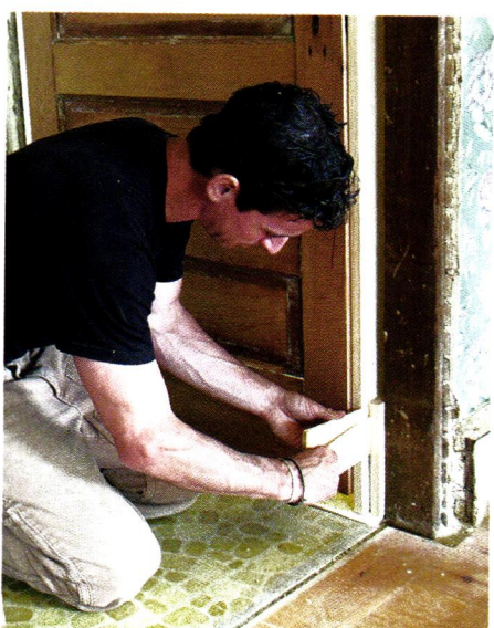
With the door jamb sitting in its new location, Mark uses a 2' level to register the assembly flush with the wall surface, then pops a nail into the top, middle, and bottom. After aligning the hinge barrels and sliding them together, Marks shims the jamb straight. Last step: Mark places a 3" deck screw through the hinge leaf and snugs it into solid framing.
