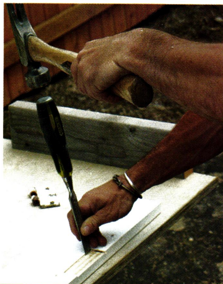
After marking the new location of the hinges, Mark uses a router and mortising jig to cut the mortises. For mortises on the jamb leg, he takes a chisel to the corners to make them nice and square. Next, he assembles the jamb, pinning it together with just a few screws so that it's ready to be moved into position, but can still be disassembled if adjustments are necessary.
