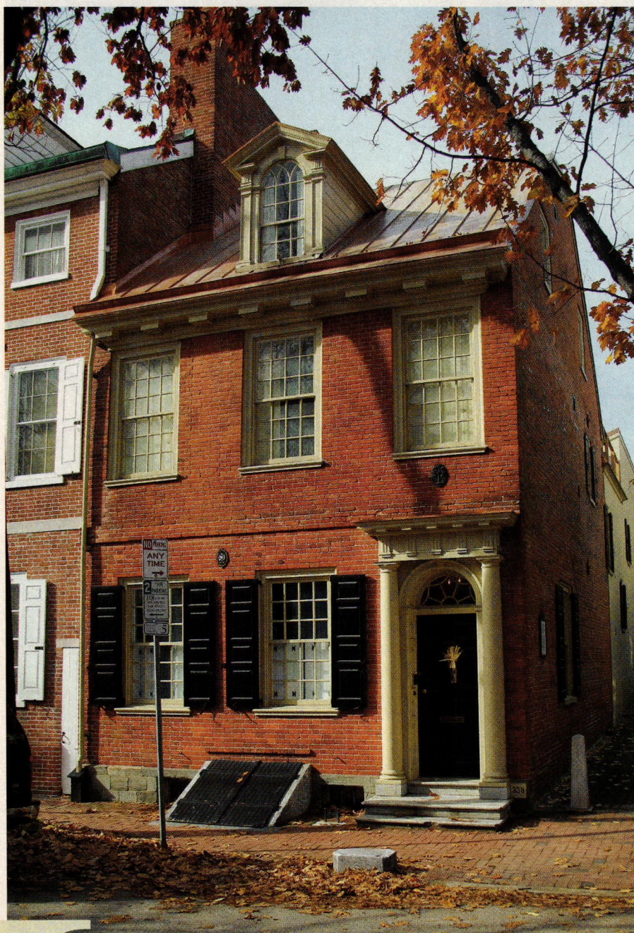
LEFT: The house that carpenter Thomas Nevel built for himself in 1770 has a decorated dormer window and an uncommon mutule cornice—good Georgian features. OPPOSITE, TOP: Rows of compatible houses build the charm of Society Hill. BOTTOM: More refined Georgian houses, like the circa 1785 Francis Hopkinson House, typically boast pedimented entries and fancy brickwork.
