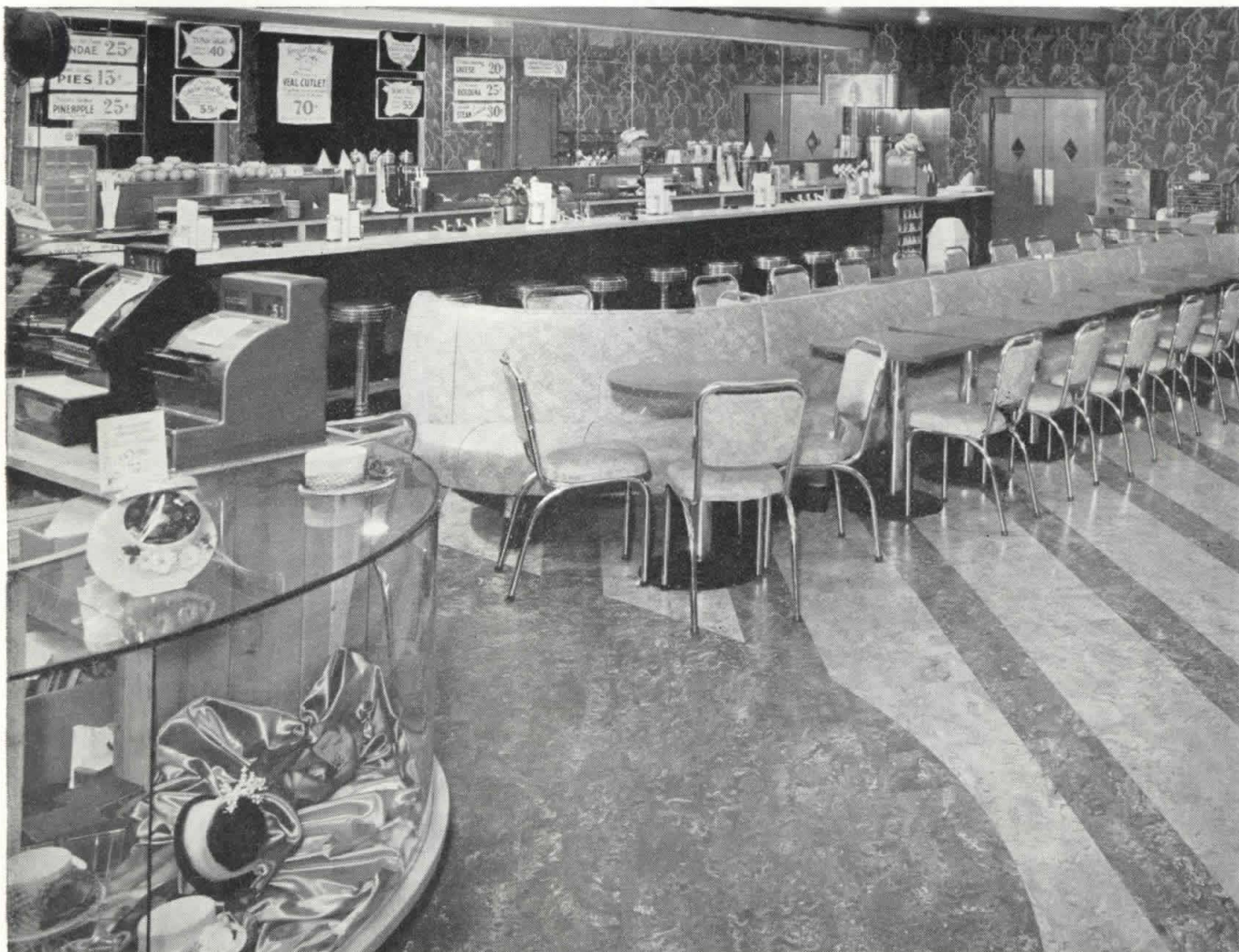
1. This beautiful floor installation in the Colonial House Candy Shop, East Orange, New Jersey, shows
