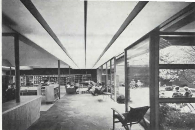
Above—luminous ceiling in reading room of Fitchburg Youth Library combines cold cathode lamps with a corrugated vinyl ceiling surface. Architects, Carl Koch and Associates. Photo: Ezra Stoller © Pictor.
