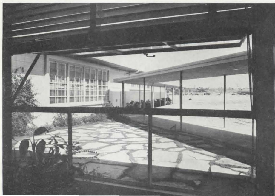
The walk connecting the lobby area and the building department wing defines a triangular, landscaped court.
