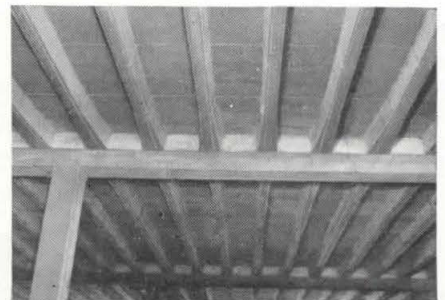
CONCRETE JOISTS eliminate much of the concrete below the neutral axis, saving money, saving material. Suited to buildings with long spans: stores, offices, apartments, hotels.
