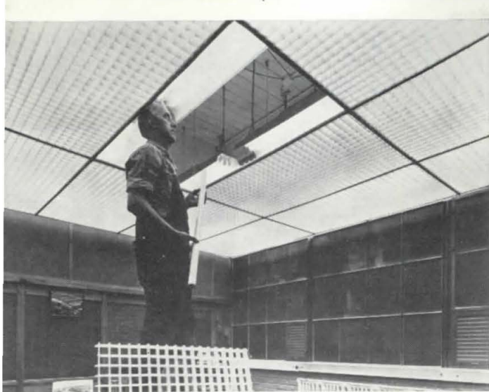
Above—luminous ceiling in reading room of Fitchburg Youth Library combines cold cathode lamps with a corrugated vinyl ceiling surface. Architects, Carl Koch and Associates. Photo: Ezra Stoller © Pictor.
