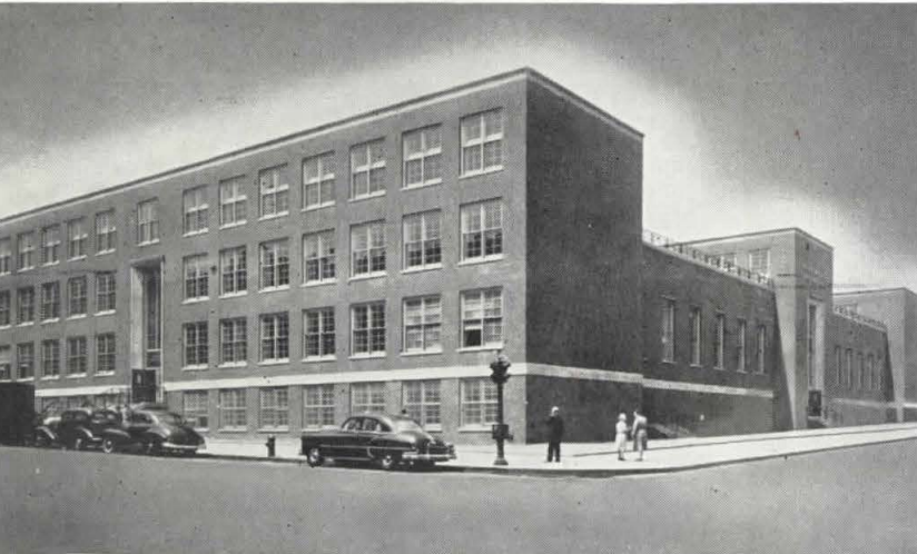
Above: Junior High School 54, Manhattan, New York City. Architect: Eric Kebbon. Engineer: T. F. Dwyer, Board of Education, City of New York. Heating Contractor: Daniel J. Rice, Inc., Long Island City, N. Y.
