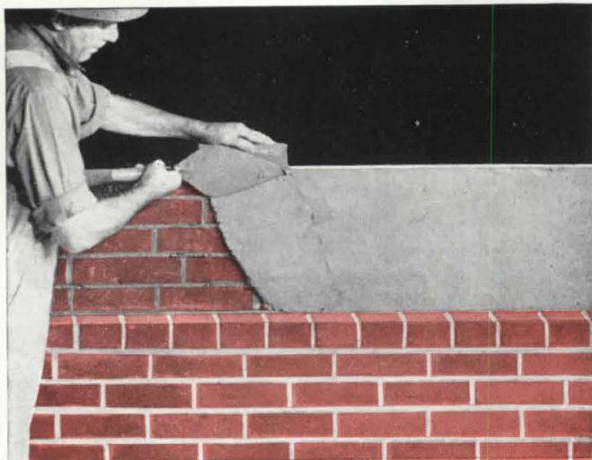
The face brick should be backplastered.
