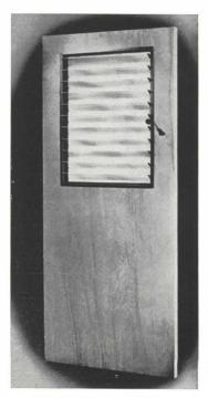
Glass-louvered Door: "Sun-Air"/ flush hardwood-plywood face/ also has rustproof-steel screen/ 1<sup>3</sup>/4" thick, 2' 8" wide, 6' 8" high/ Davidson Plywood & Lumber Co., 3631 E. Washington Blvd., Los Angeles 23, Calif.
