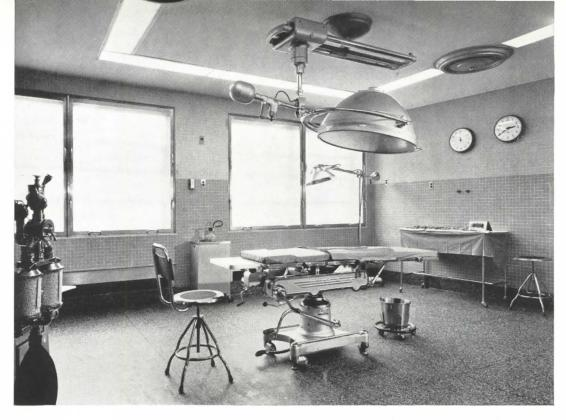
Typical of all operating rooms, the one shown (above) is fully air conditioned and has walls of ceramic mosaic tile to facilitate cleaning. Conductive terrazzo floors provide controlled drain-off of static charges. The rooms receive daylight, but to maintain temperature and humidity conditions there are inner glass screens, with temperature air streams creating a pressurized barrier, to prevent dust infiltration.
