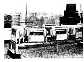
Eight electrical "watchdogs" installed on the roof of the new Los Angeles Statler Center hotel and office building automatically vary the cooling capacities of the building's air-conditioning system according to changes in the angle and intensity of the sun's rays. Each unit of the solar compensator faces a direction corresponding to one of the major exposures of the building's wings. Carrier Corp., Svracuse, N. Y.
