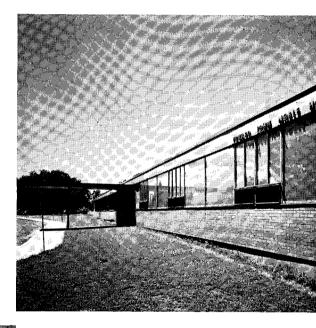
Both the one-story, southeast front, and the two-story side facing the river are lined with continuous windows, made up of alternating fixed and operable units.
