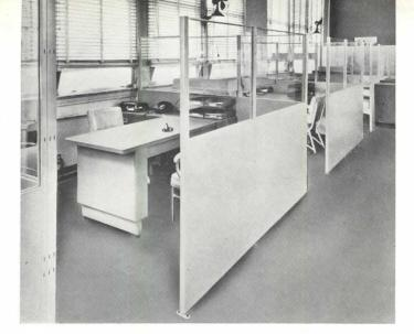
Free-Standing Partitions: supported by floor connector of heavy-metal angle that fits inside partition post/ broad base slotted to adjust for uneven floors may be attached to floor/ clamp grips and holds adjoining panels/ The Globe-Wernicke Co., Ross & Carthage Ave., Cincinnati 12, Ohio
