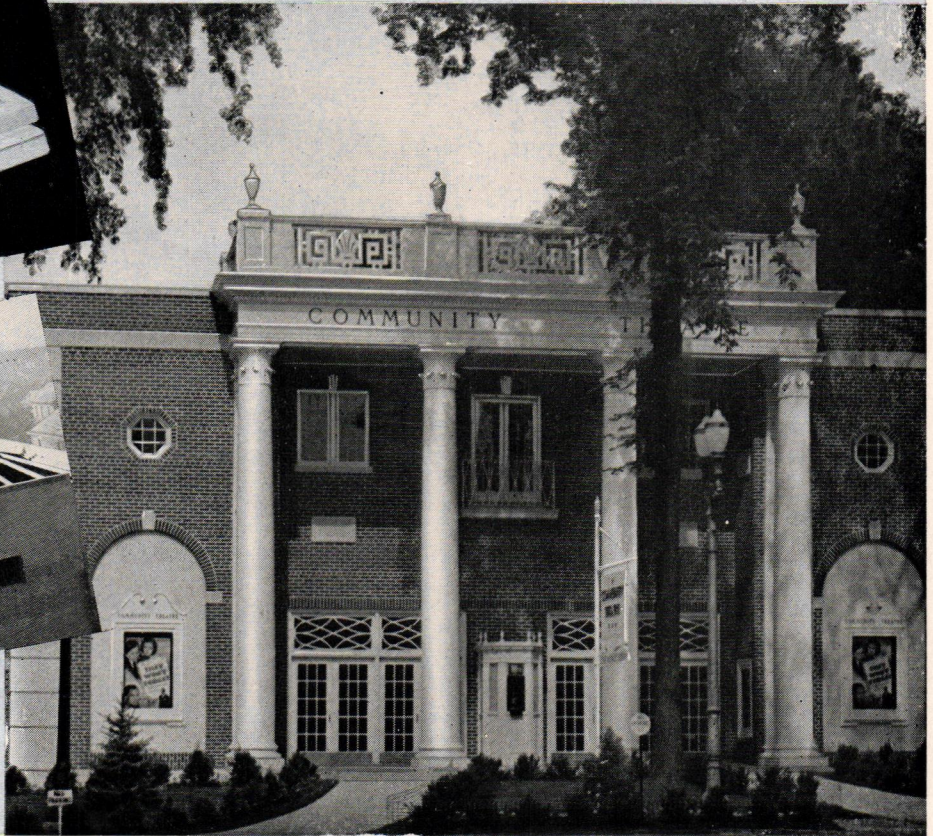
The Community Theatre at Saratoga Springs, N. Y., designed by Thomas W. Lamb, New York, is one of several in the American Theatres Corporation in which Plank roof-decks are installed.
