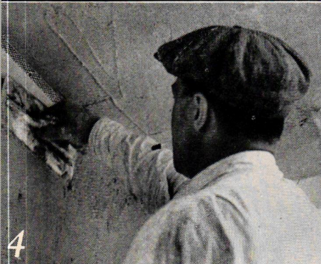
4 Providing both insulation and plaster base in one product. Note joint reinforcement.
