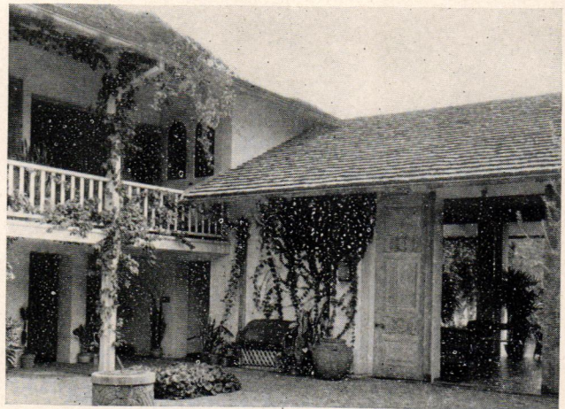
A two-story porch gives circulation in the Balding house
