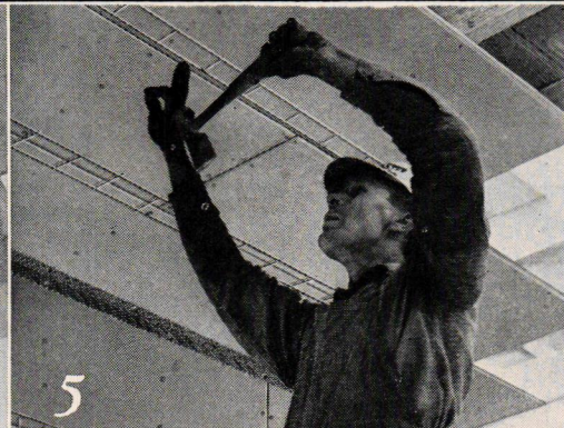
5 Sheets span 3 studs—yet one man handles easily.
