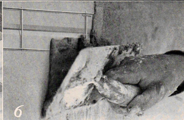
6 Exclusive USG reinforcing to minimize plaster cracks.
