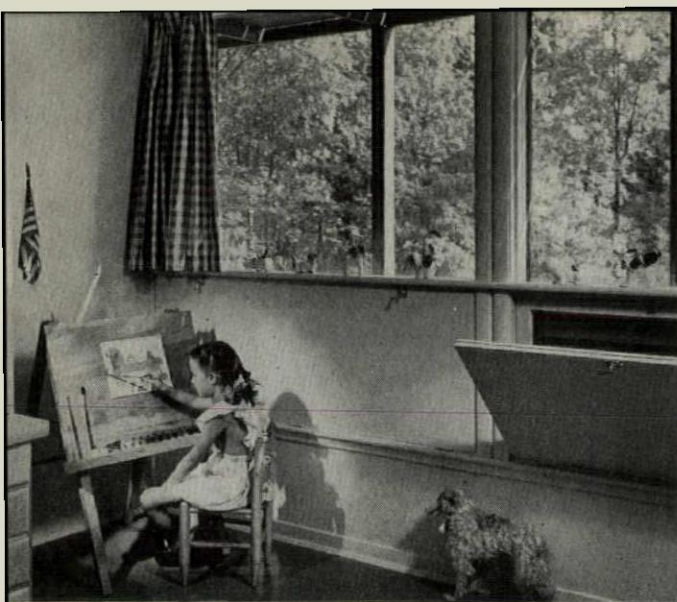
Fixed windows, of three thicknesses of heat-resisting glass with air spaces between, make it possible to use great expanses of glass even in northern latitudes. For ventilation, George Fred Keck, Chicago architect, provides louvers below with inside, bottom-hinged doors. Above, interior with ventilator open; below, ventilator closed, and view from outside.
