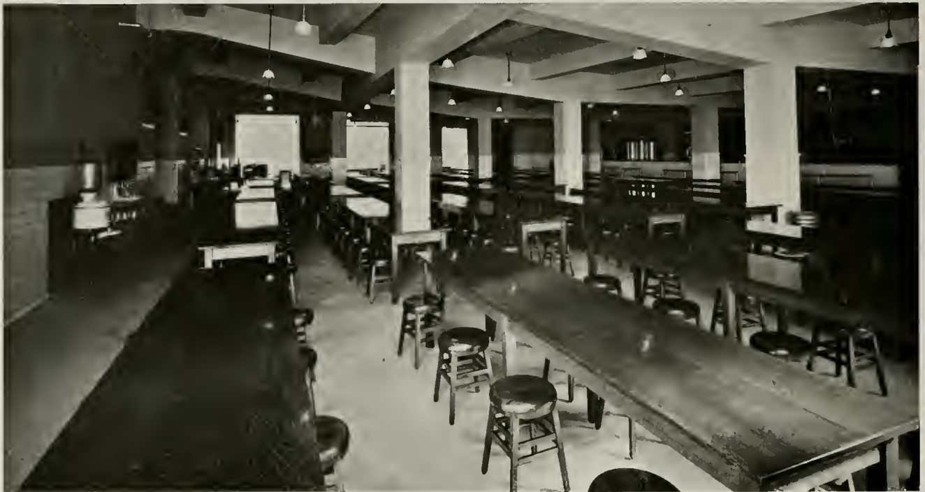
LUNCH ROOM, GROVER CLEVELAND HIGH SCHOOL WM. B. ITTNER, ARCHITECT
