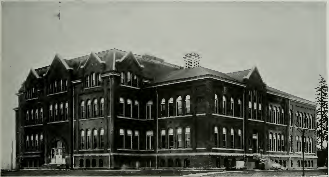
WHITMORE SCHOOL, TACOMA, WASHINGTON ROOFER EDWARD MILLER CORNICE & ROOFING CO
