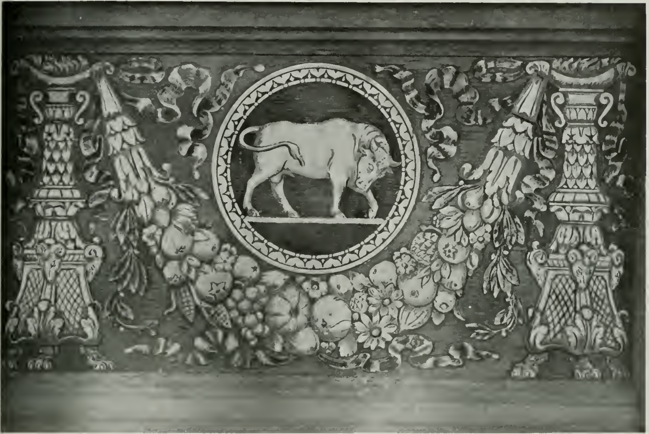
One of Ten Typical Three-Color Sgraffito Panels in Main Facade, Hilgard Hall, University of California
