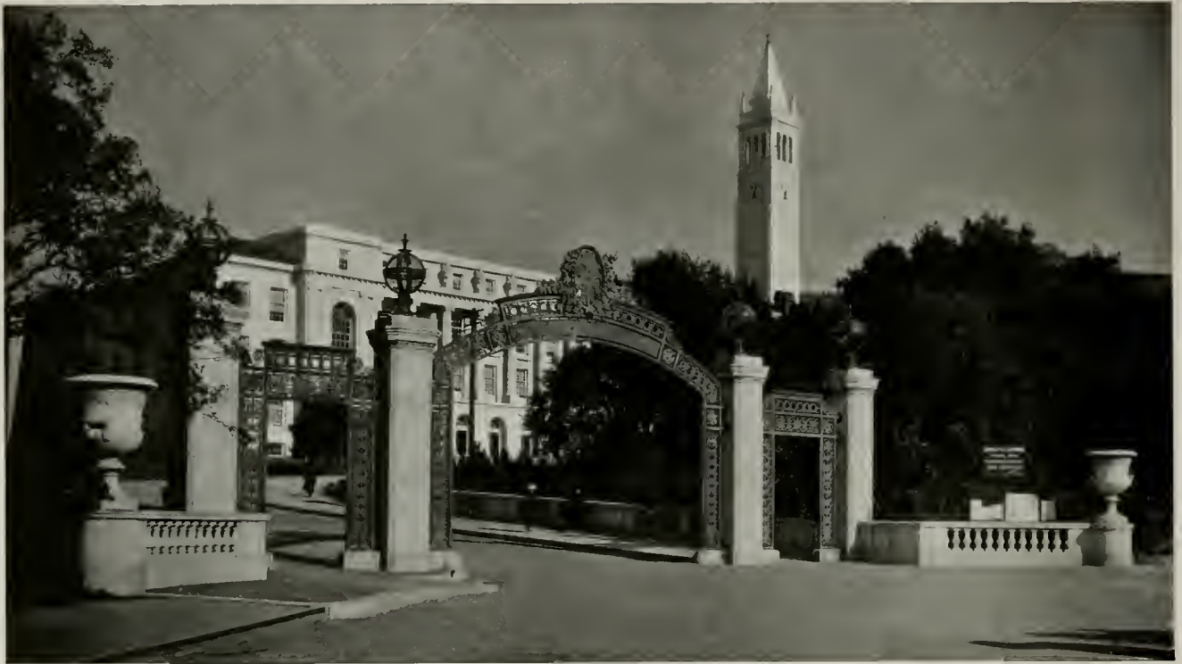
THE SATHER GATE, UNIVERSITY OF CALIFORNIA JOHN GALEN HOWARD, ARCHITECT
