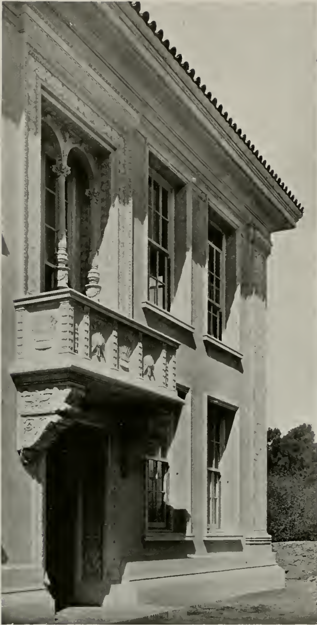
Northeast Balcony and Entrance with Sgraffito Borders and Reveals, Hilgard Hall, University of California
