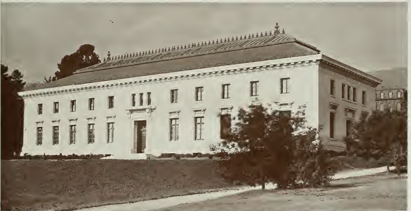
CALIFORNIA HALL UNIVERSITY OF CALIFORNIA JOHN GALEN HOWARD, ARCHITECT
