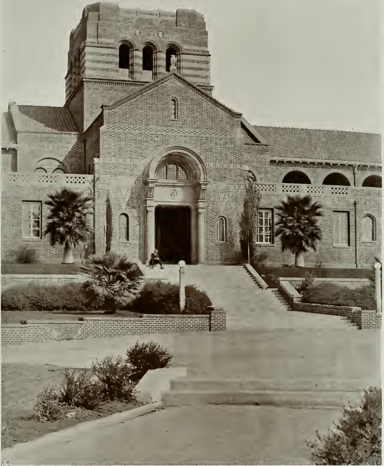
ENTRANCE DETAIL, SANTA MONICA HIGH SCHOOL, SANTA MONICA, CAL. ALLISON AND ALLISON, Architects
