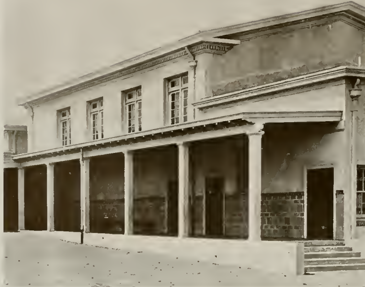
View Showing Covered Play Space, McKinley Elementary School, San Leandro, Cal. JOHN J. DONOVAN, Architect
