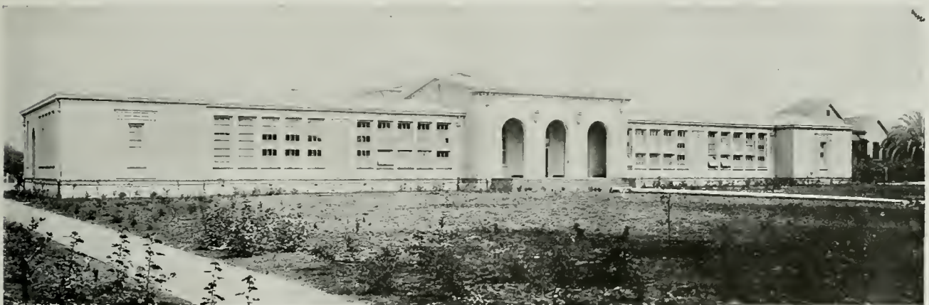
FRONT ELEVATION, MCKINLEY ELEMENTARY SCHOOL, SAN LEANDRO, CAL. JOHN J. DONOVAN, ARCHITECT
