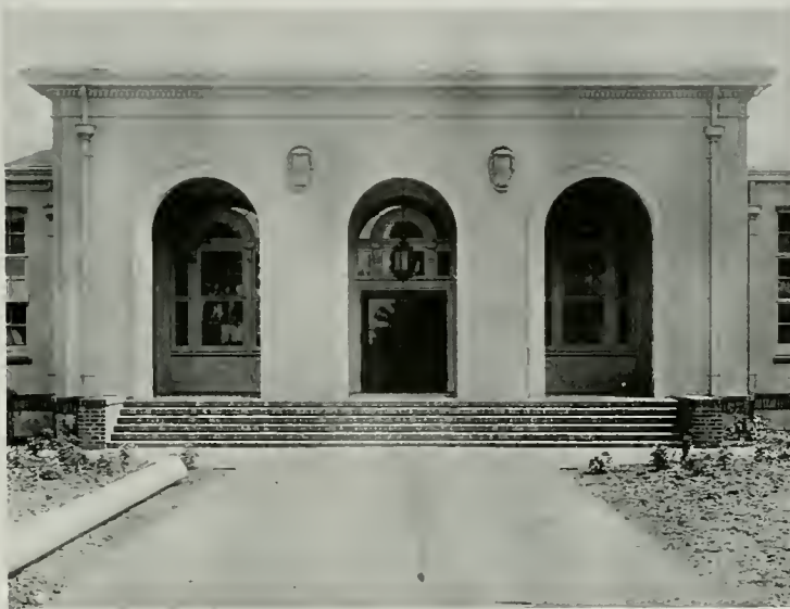
MAIN ENTRANCE, MCKINLEY ELEMENTARY SCHOOL, SAN LEANDRO, CAL. JOHN J. DONOVAN ARCHITECT
