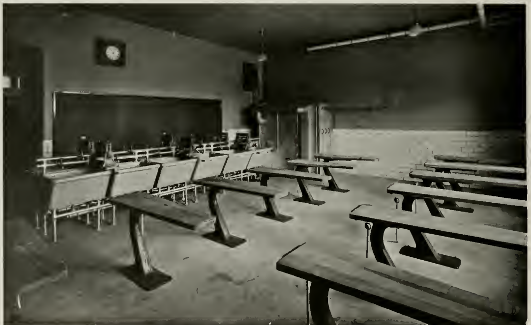
LAUNDRY, GROVER CLEVELAND HIGH SCHOOL WM. B. ITTNER, Architect
