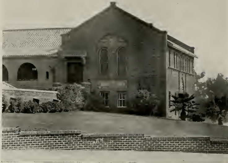
End of Science and Household Arts Building Santa Monica High School, Santa Monica, Cal. ALLISON AND ALLISON, Architects
