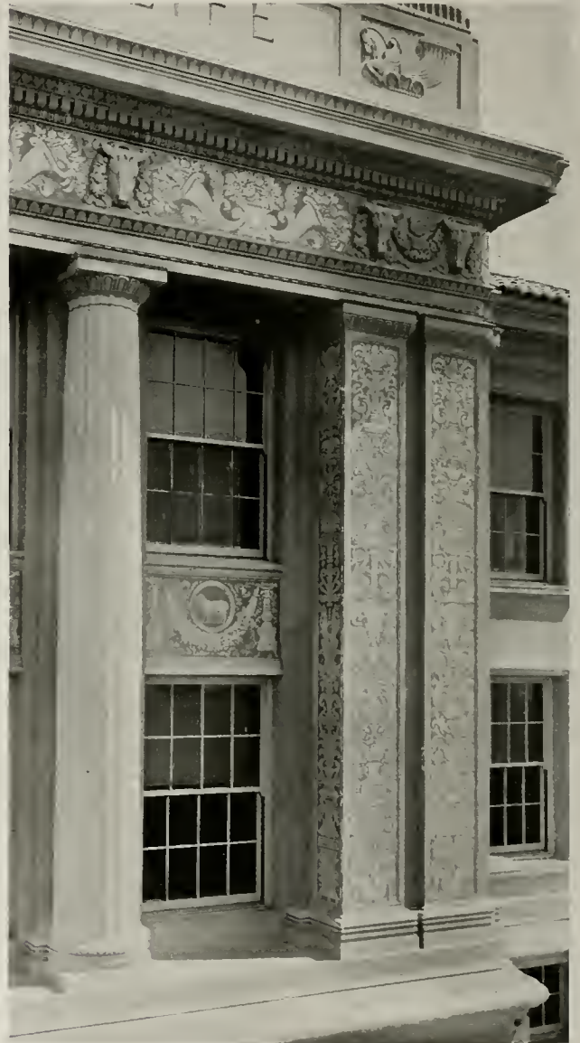
Typical Detail of Main Facade Showing Extensive Sgraffito Treatment, Hilgard Hall, University of California
