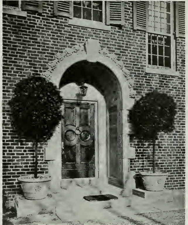
Detail of Modern Doorway. Howard Shaw, Architect
