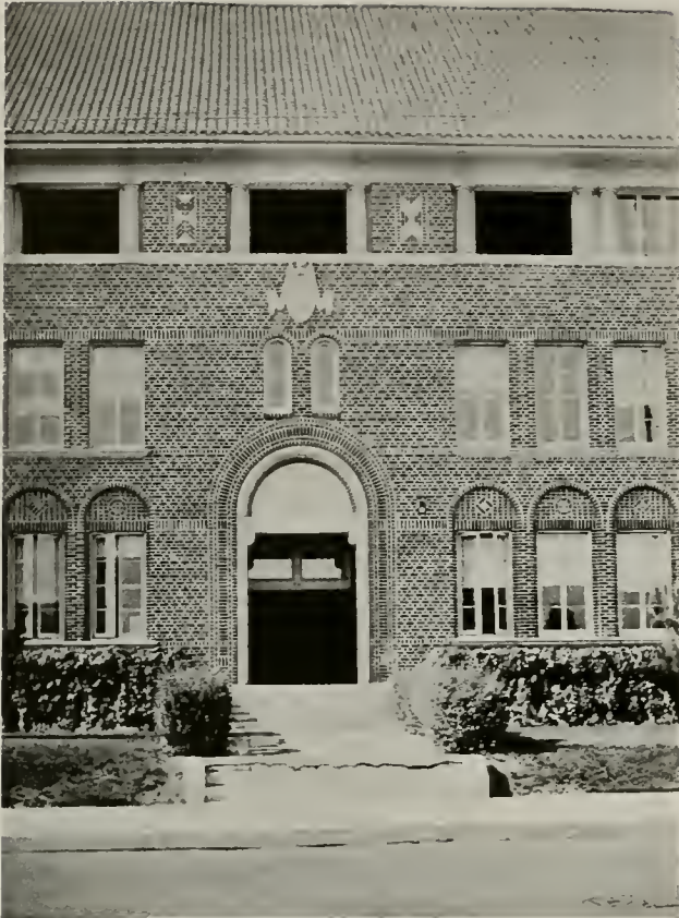
Entrance Detail, High School, Wilmington District, Los Angeles, Cal. ALLISON AND ALLISON Architects
