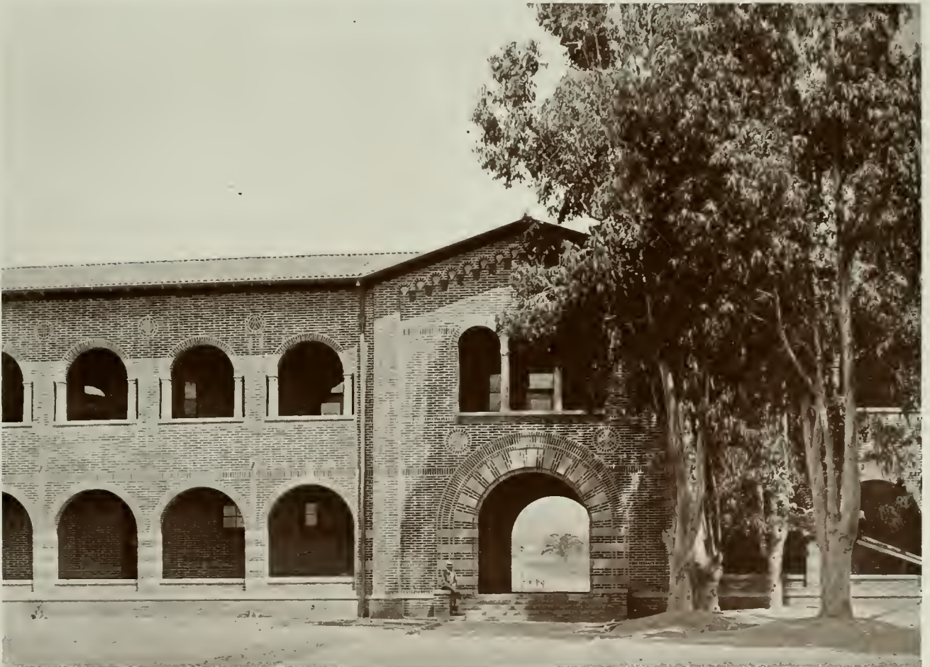
DETAIL, TRAINING SCHOOL FORECOURT LOS ANGELES STATE NORMAL SCHOOL, LOS ANGELES, CAL. ALLISON AND ALLISON, Architects
