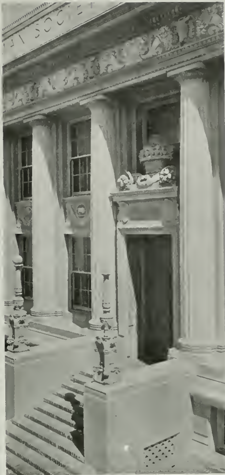
Main Entrance Detail with Sgraffito Frieze Above and Symbol Panels, Etc., Hilgard Hall, University of California
