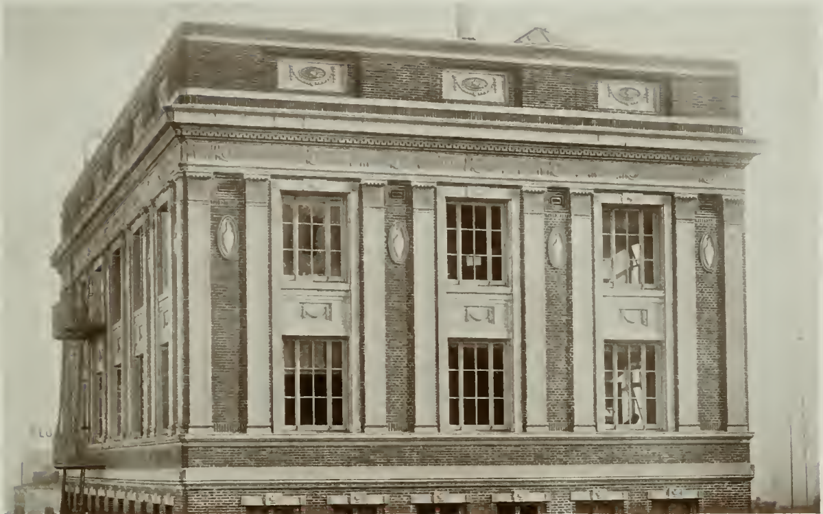
DETAIL OF UPPER STORIES
