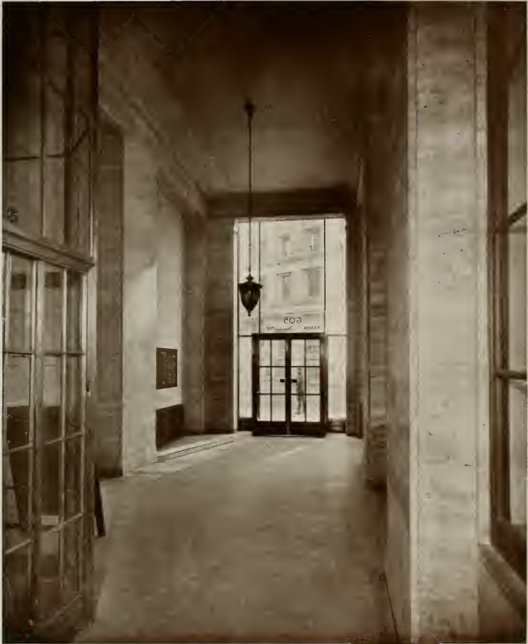
ENTRANCE LOBBY TO OFFICES, SANTA FE BUILDING, SAN FRANCISCO WOOD & SIMPSON, ARCHITECTS
