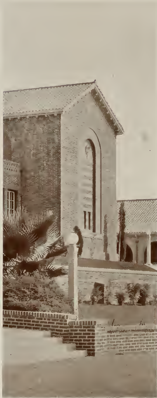
End Pavilion Santa Monica High School, Santa Monica, Cal. ALLISON AND ALLISON Architects
