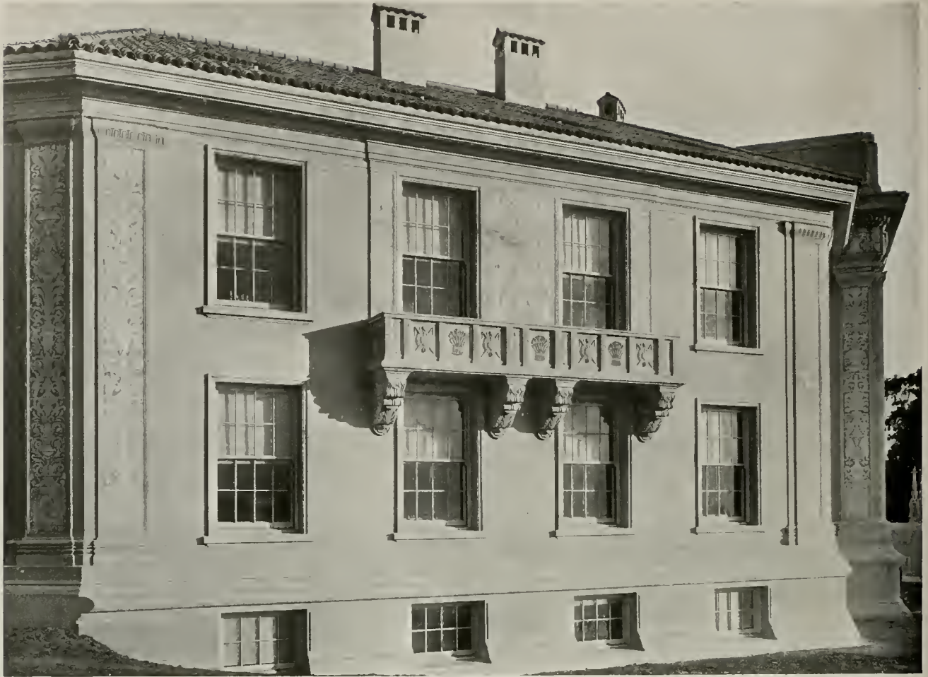
Northwest Balcony Showing Sgraffito Panels and Pilasters, Hilgard Hall, University of California
