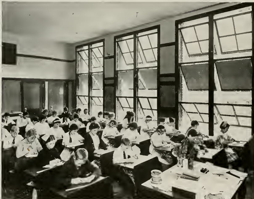
TYPICAL INTERIOR OF CLASS ROOM
