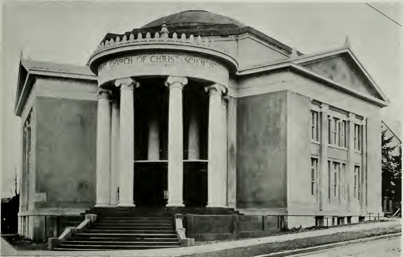
E. MILLER CORNICE & ROOFING CO Roofers
