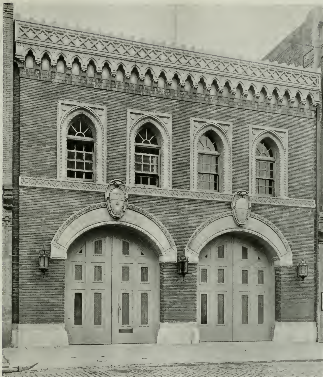
SAN FRANCISCO FIRE DEPARTMENT - ENGINE No. 4
