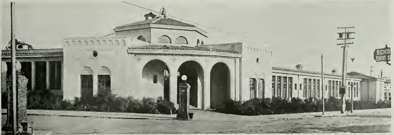
CLAREMONT ELEMENTARY SCHOOL, OAKLAND, CAL. JOHN J. DONOVAN AND W. D. REED, ASSOCIATE ARCHITECTS
