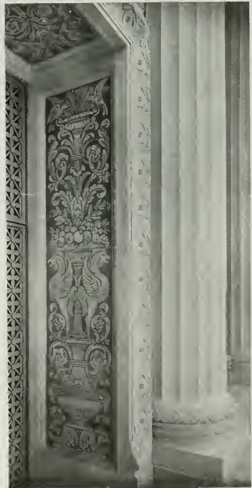
Jamb Detail of Main Entrance Showing Sgraffito Treatment, Hilgard Hall, University of California
