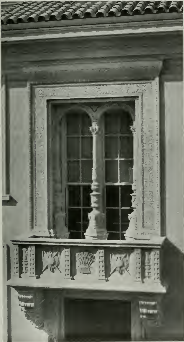
Southeast Balcony Detail with Sgraffito Treatment to Border and Reveals. Hilgard Hall, University of California
