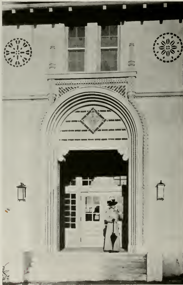
Entrance Detail, Grammar School, Holtville, Cal. ALLISON AND ALLISON Architects
