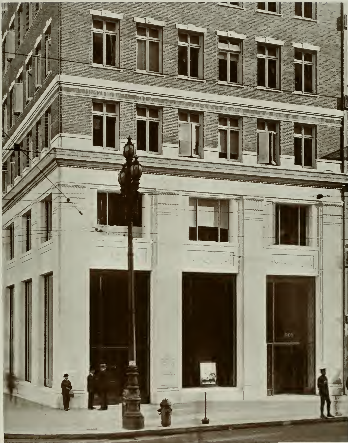
DETAIL OF LOWER STORIES, SANTA FE BUILDING, SAN FRANCISCO WOOD & SIMPSON ARCHITECTS
