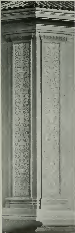
Typical Main Pilasters Showing Sgraffito Detail, Hilgard Hall, University of California
