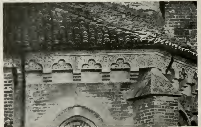
Cornice in Chapel, Vercelli.
