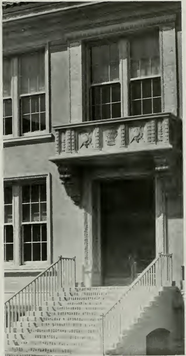
East Middle Entrance and Balcony Showing Sgraffito in Jambs and Borders. Hilgard Hall, University of California
