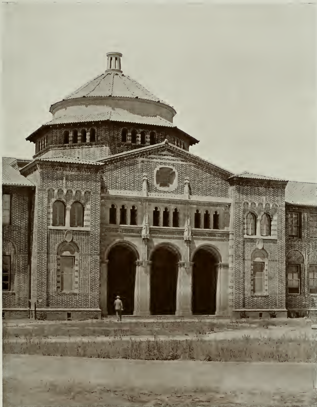
DETAIL MAIN ENTRANCE ADMINISTRATION BUILDING, LOS ANGELES STATE NORMAL SCHOOL ALLISON AND ALLISON Architects
