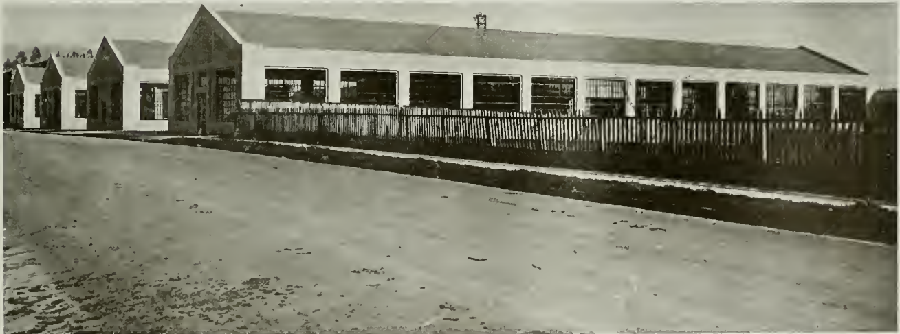
NORTH VIEW OF SHOPS
