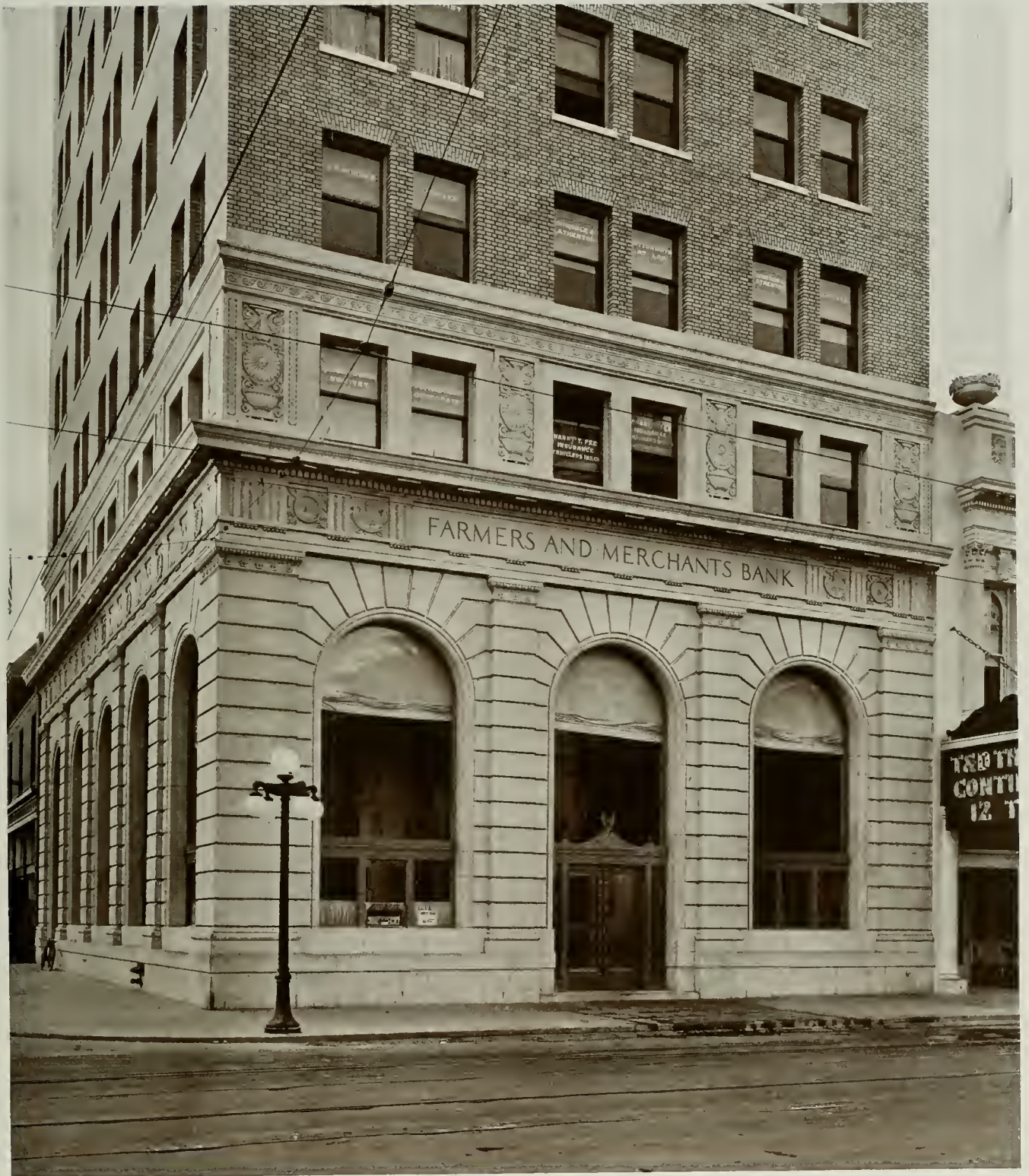
DETAIL OF LOWER STORIES, FARMERS AND MERCHANTS BANK, STOCKTON, CAL. GEORGE W. KELHAM, ARCHITECT
