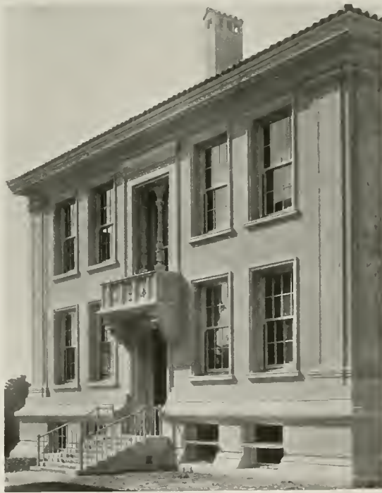
Southeast Balcony, with Sgraffito Borders, Jambs and Pilasters, Hilgard Hall, University of California.
