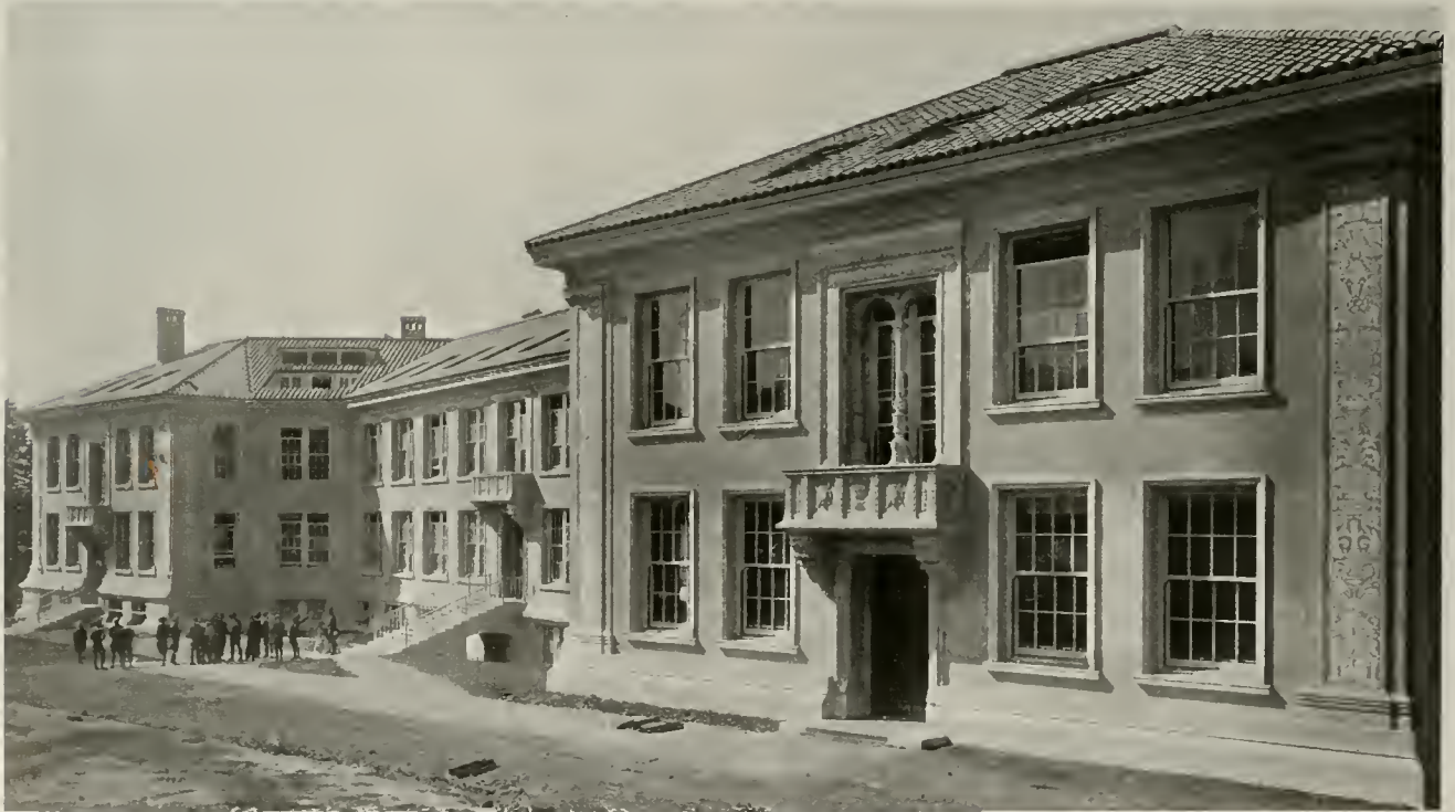
Rear Elevation of Hilgard Hall, University of California JOHN GALEN HOWARD, Architect
