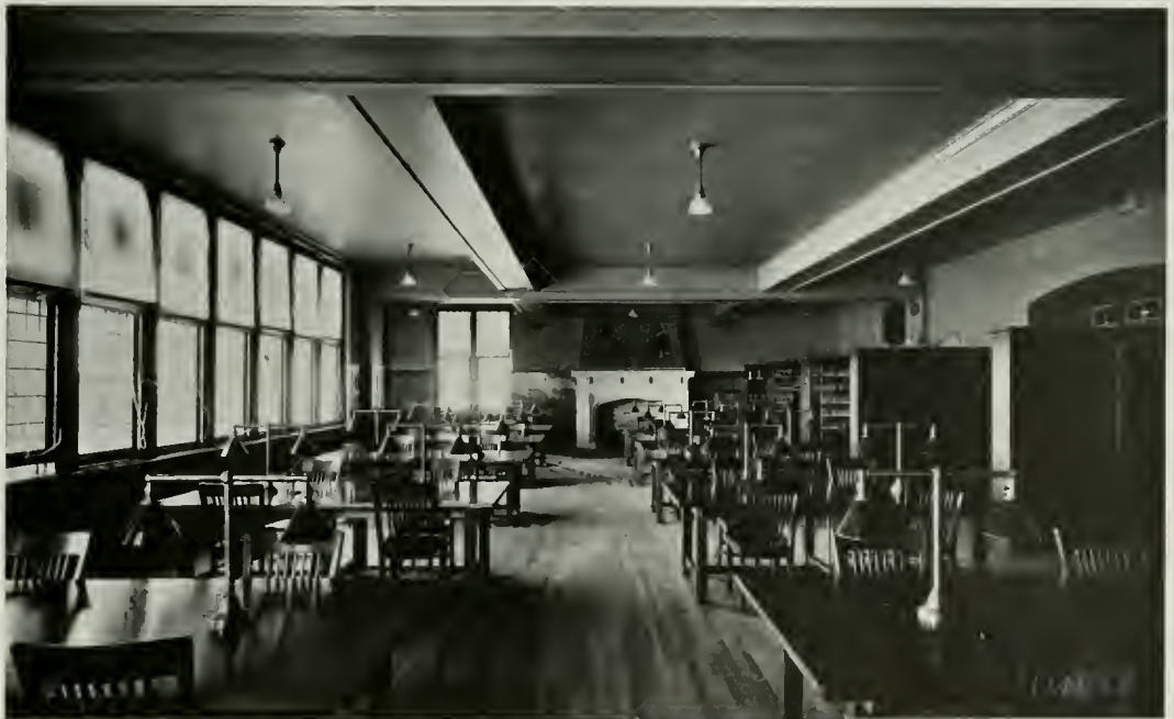
LIBRARY, GROVER, CLEVELAND HIGH SCHOOL WM. B. ITTNER, Architect
