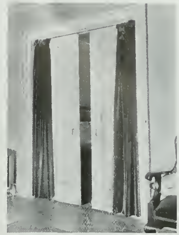
Pitcher's Sliding Doors Installed
