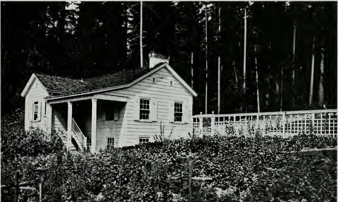
LAUNDRY AND SERVANTS' QUARTERS FROM PATH TO GARAGE RESIDENCE OF L. D. LEWIS, HIGHLANDS, NEAR SEATTLE, WASH. W. R. B. WILLCOX, Architect
