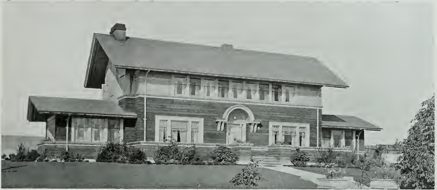
RESIDENCE OF J. C. BLACK, SEATTLE, WASH. ANDREW C. P. WILLATZEN, Architect
