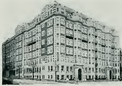
THE BRAEMORE, Boston BLACKHALL, CLAPP & WHITMORE, Architects MEYER MELTZER, Plumber 431 "Standard" Fixtures
