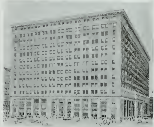
Railway Building, St. Paul, Minn., in which 1000 Perennial Shades are installed.
