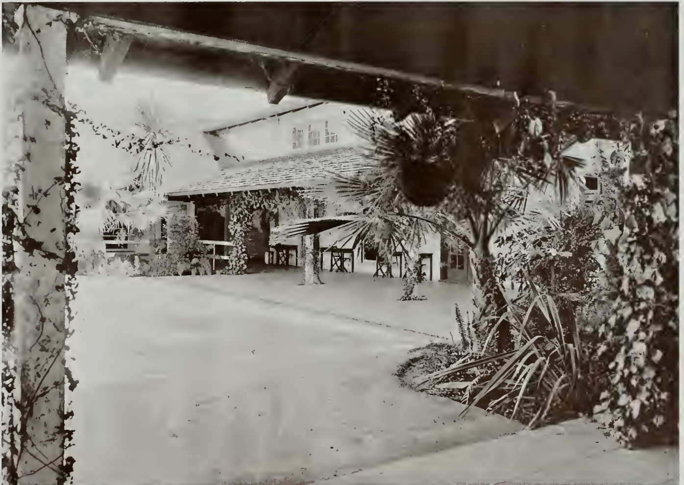
VIEWS IN PATIO POLYTECHNIC ELEMENTARY SCHOOL, PASADENA, CAL. MYRON HUNT AND ELMER GREY, Architects
