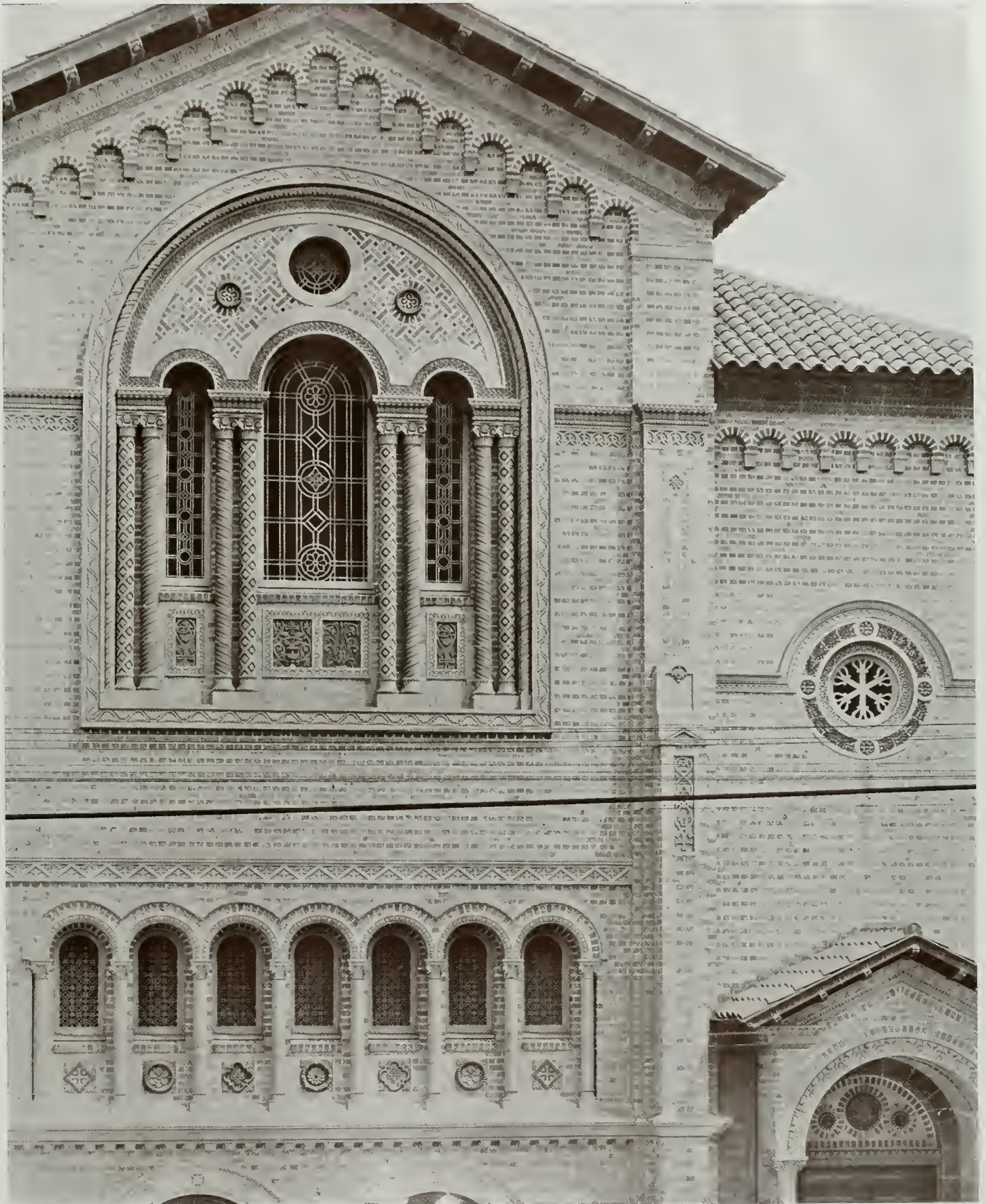
DETAIL UPPER PORTION OF FRONT THIRD CHURCH OF CHRIST SCIENTIST, SAN FRANCISCO, CAL. EDGAR A. MATHEWS, Architect
