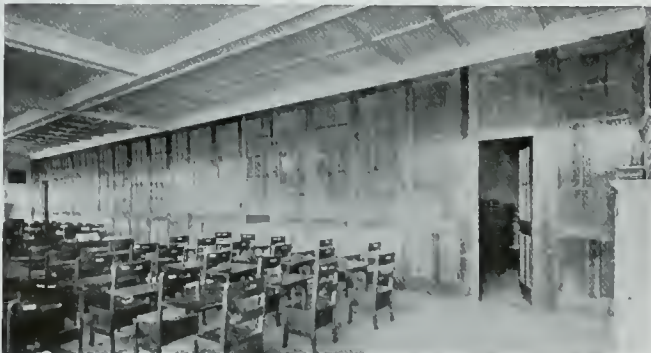
SHOWING SAME PARTITION AS ABOVE DRAWN This partition, installed in a public school auditorium, is 12 feet high and 72 feet long. Note the glass panels and shuttle doors.
