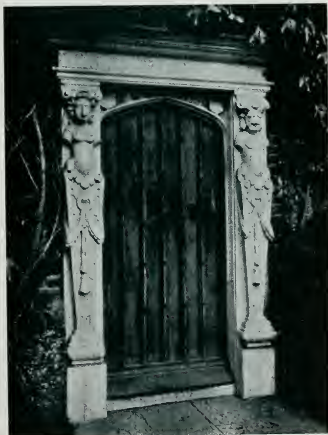
ENTRANCE DOORWAY TO WELL HOUSE
