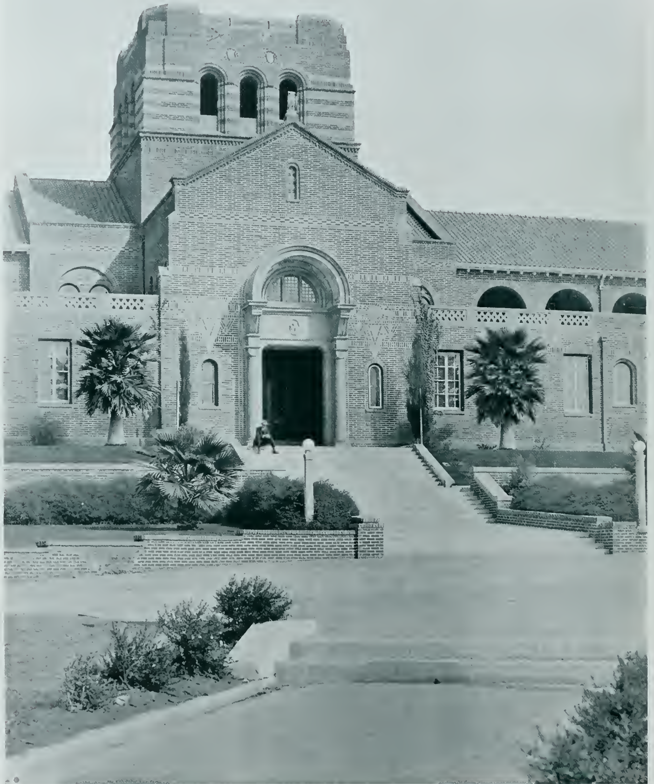
ENTRANCE DETAIL. SANTA MONICA HIGH SCHOOL, SANTA MONICA, CAL
