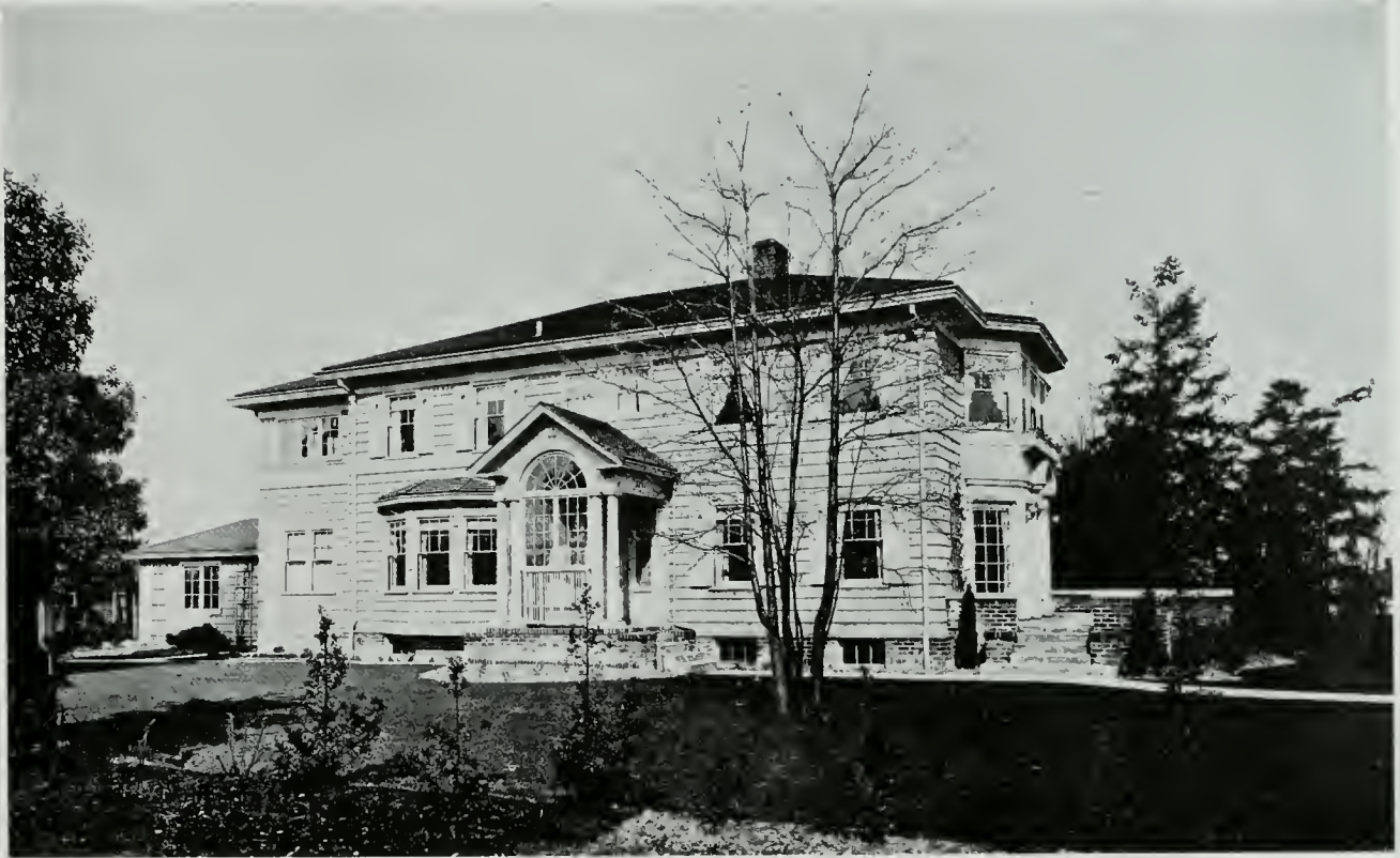
RESIDENCE OF WILLIAM G. JOHN, SEATTLE, WASH. ARTHUR L. LOVELESS, Architect
