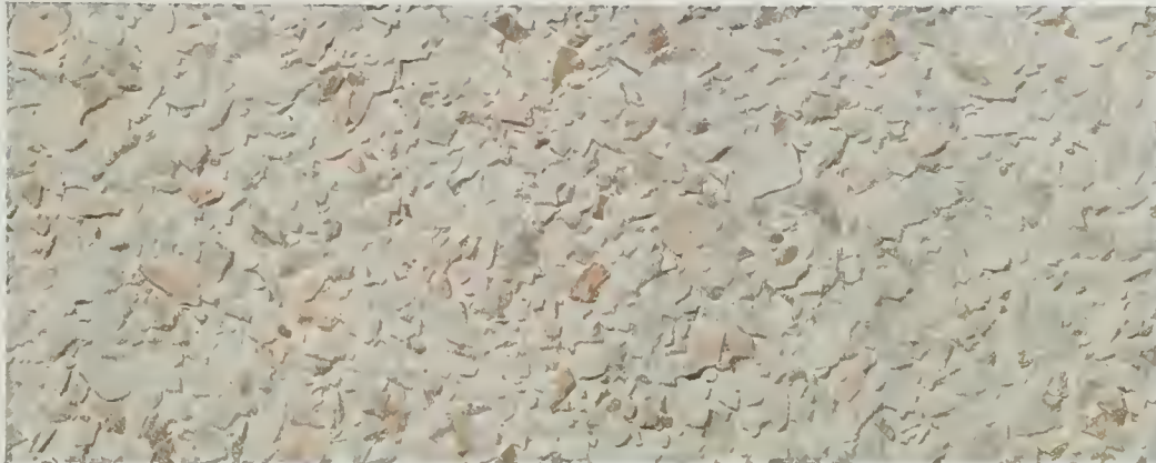
Hunt House formula: 1 part Atlas-White Cement; 1 part white quartz and pink felspar dust. While plastic, 1 part quartz and 3 parts felspar, \frac{1}{4} -inch grits thrown on and lightly floated.
