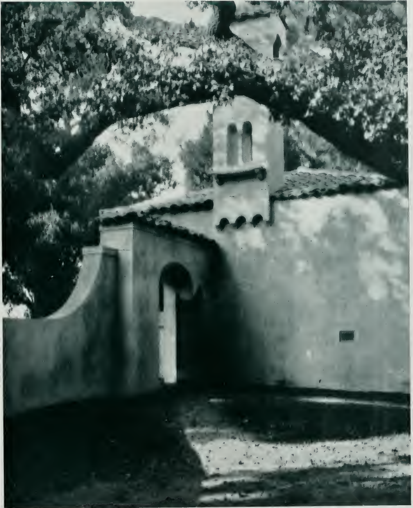
GATEWAY FROM KITCHEN YARD TO WEST GARDEN HOUSE FOR CHARLES D. BLANEY, SARATOGA, CAL. WILLIS POLK & CO., Architects
