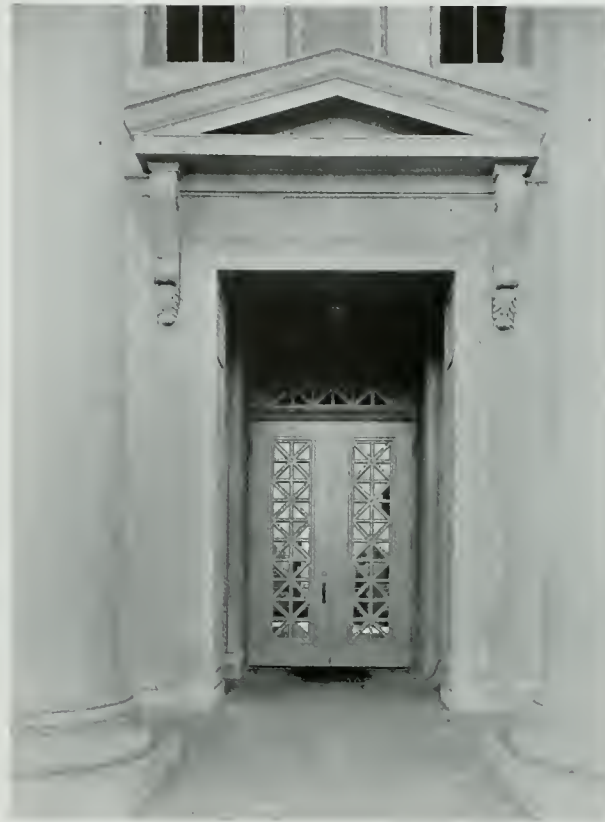
Entrance Administration Building, Polytechnic High School, Santa Ana, Cal. WITHEY & DAVIS, Architects
