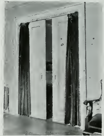
Pitcher's Sliding Doors Installed
