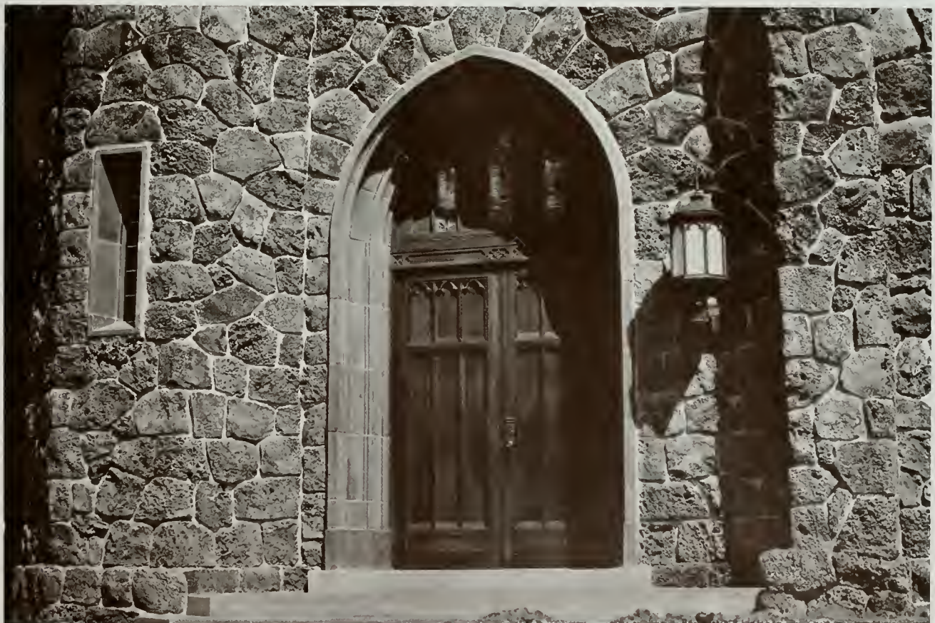
DETAIL OF ENTRANCE
