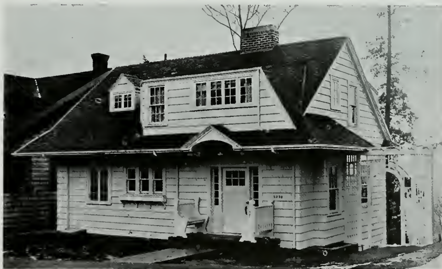
RESIDENCE OF MRS. HENRY ANGERS, SEATTLE, WASH. E. J. IVY, Architect
