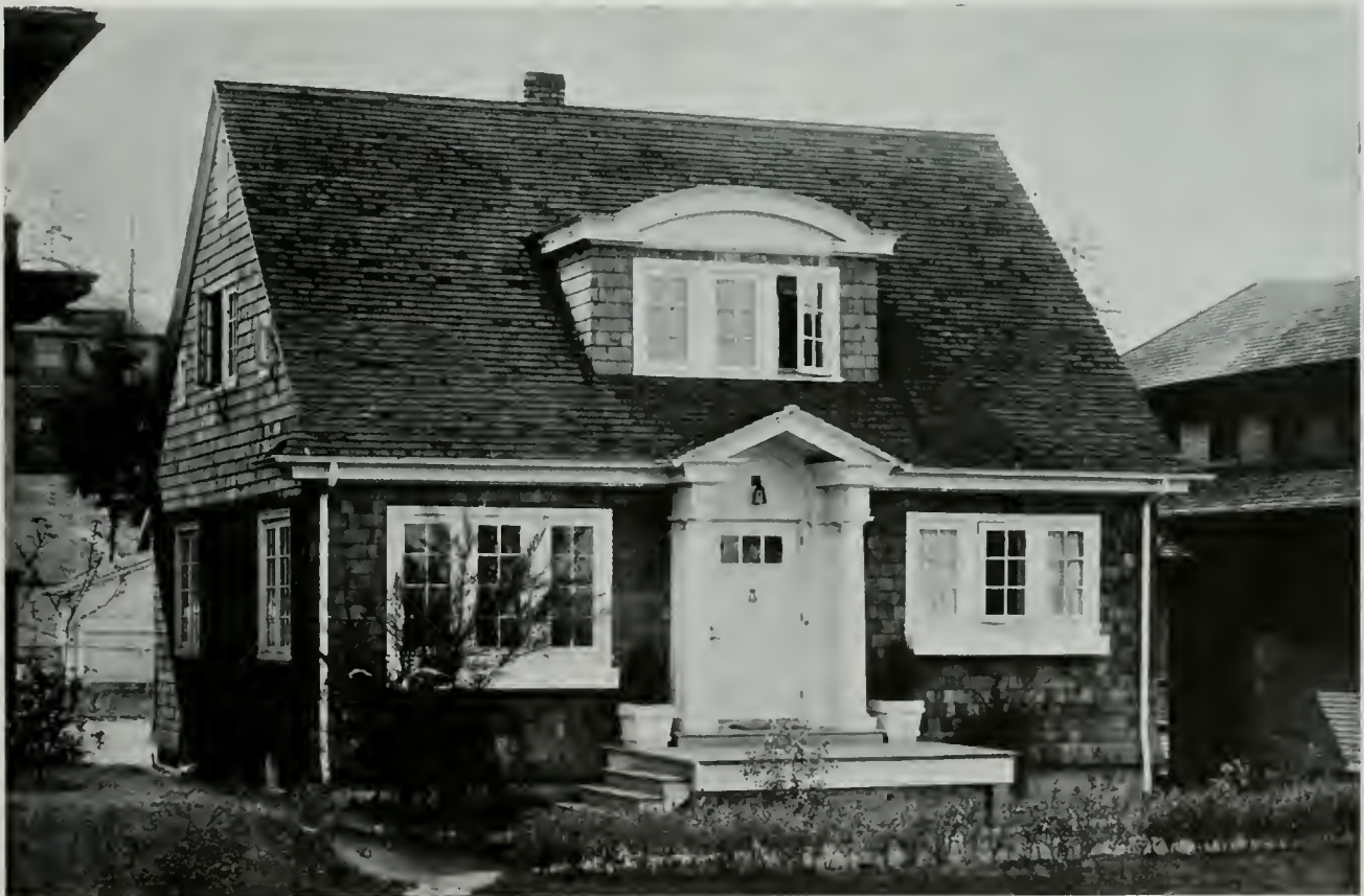
RESIDENCE OF H. H. WOLFE, SEATTLE, WASH. W. R. B. WILLCOX, Architect
