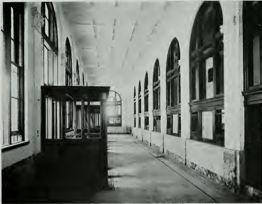
Inside Main Lobby, Looking East, United States Postoffice, Berkeley, Cal. Oscar Wenderoth, Supervising Architect
