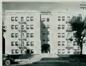
GEORGELE APARTMENTS, Los Angeles Plans by Owner, GEO. L. LOVEJOY W. A. DIEI, Plumber 235 "Standard" Fixtures
