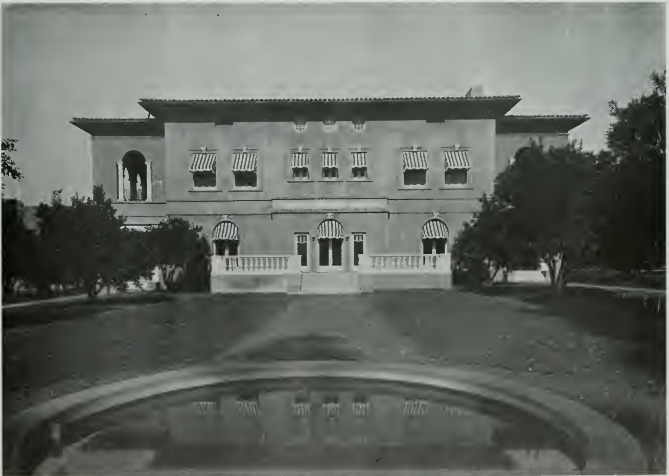
HOUSE FOR DR. ARNO BEHR, SOUTH PASADENA, CAL. REGINALD D. JOHNSON, Architect
