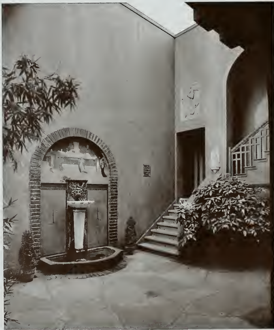
DETAIL IN COURTYARD THE PRINT ROOMS OF HILL TOLLERTON, SAN FRANCISCO WILLIAM C. HAYS, Architect
