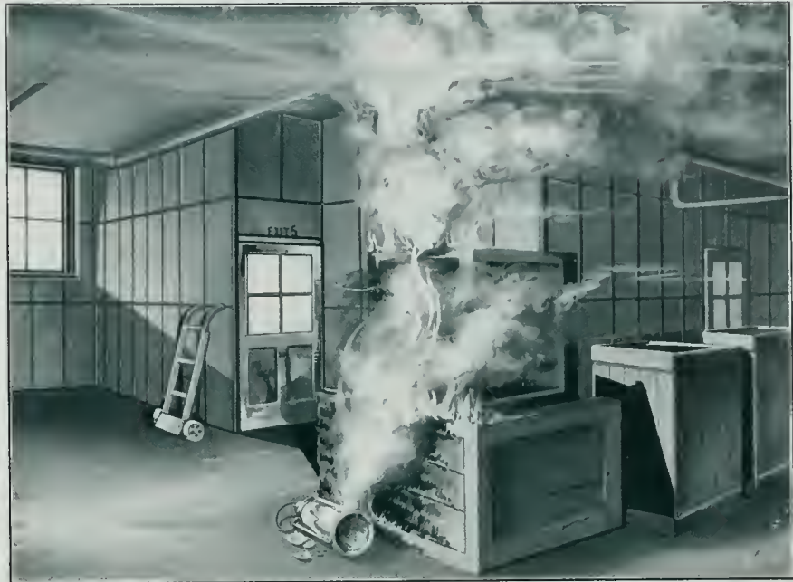
AMBLER ASBESTOS BUILDING LUMBER
