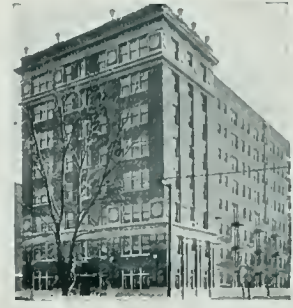
WESTMORELAND APARTMENTS HOTEL St. Louis P. J. BRADSHAW, Architect A. J. FISCHER, Plumber 253 "Standard" Fixtures
