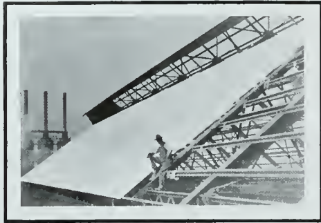
ASB*STOS CORRUGATED ROOFING BEING APPLIED
