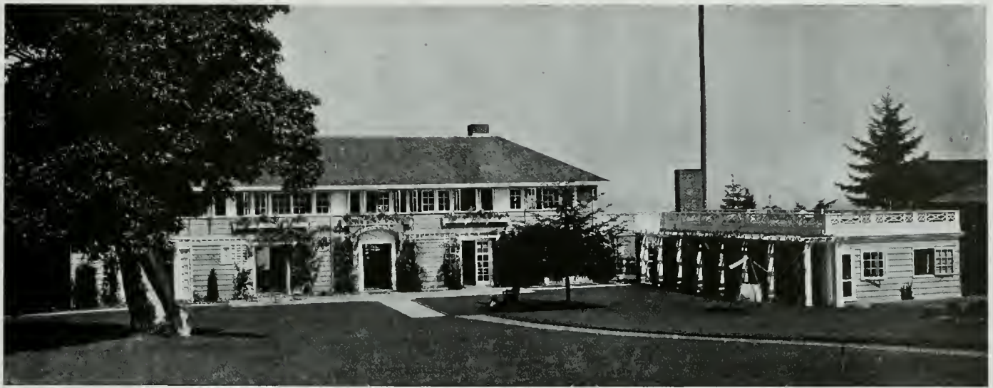
RESIDENCE OF ALEXANDER F. McEWAN, COUNTRY CLUB, BAINBRIDGE ISLAND, WASH. CARL F. GOULD, Architect
