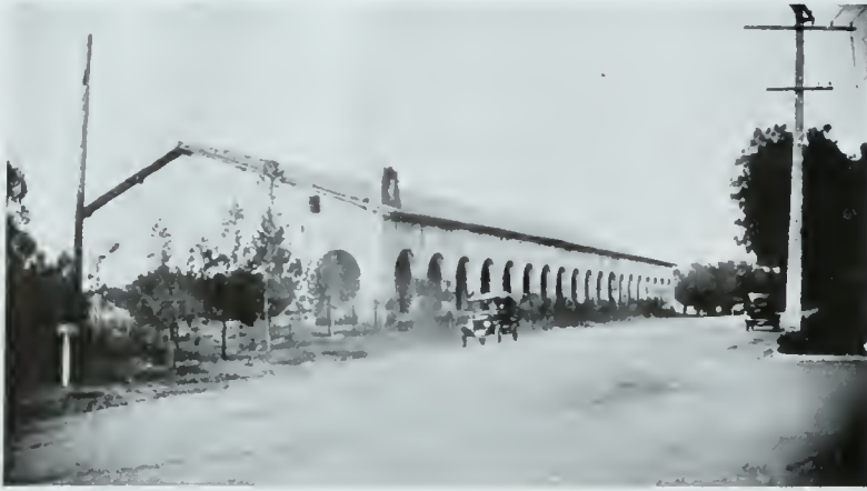
San Fernando Cloister
