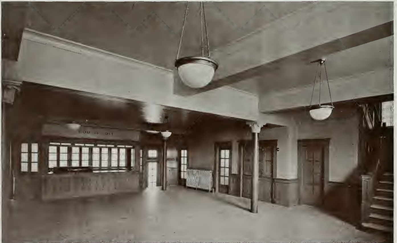
LOWER VESTIBULE OR LOBBY. VIEW TOWARDS DOORS INTO SUNDAY SCHOOL ROOM
