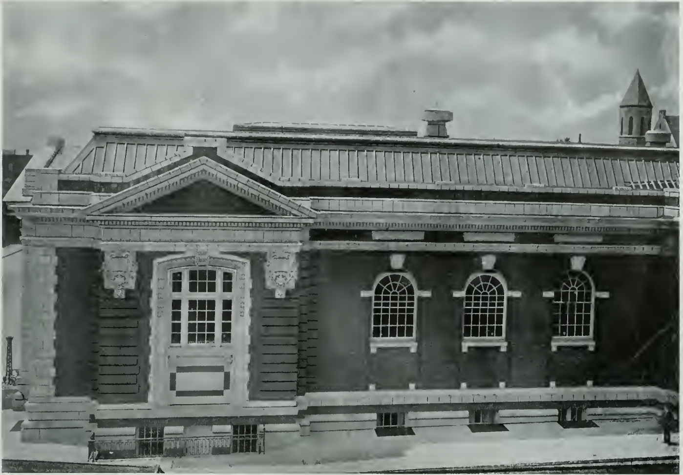
The Carnegie Library, at Frankford, Philadelphia. The tin has been laid over half-round strips to give the desired ribbed effect.
