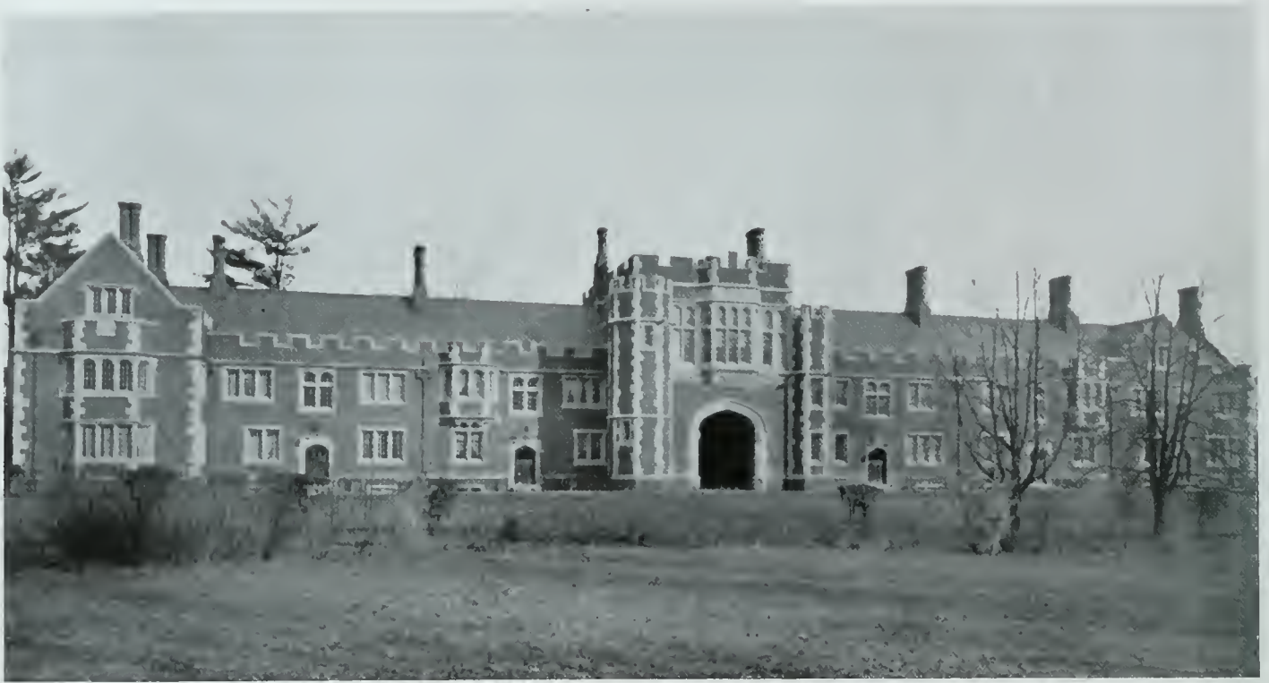
'79 HALL, PRINCETON UNIVERSITY, from "Architecture" BENIAMIN W. MORRIS, Architect
