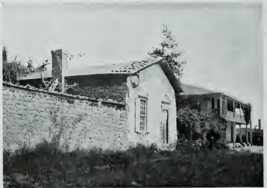
Council Larkins House and Hall of Records when Monterey was California's Capitol
