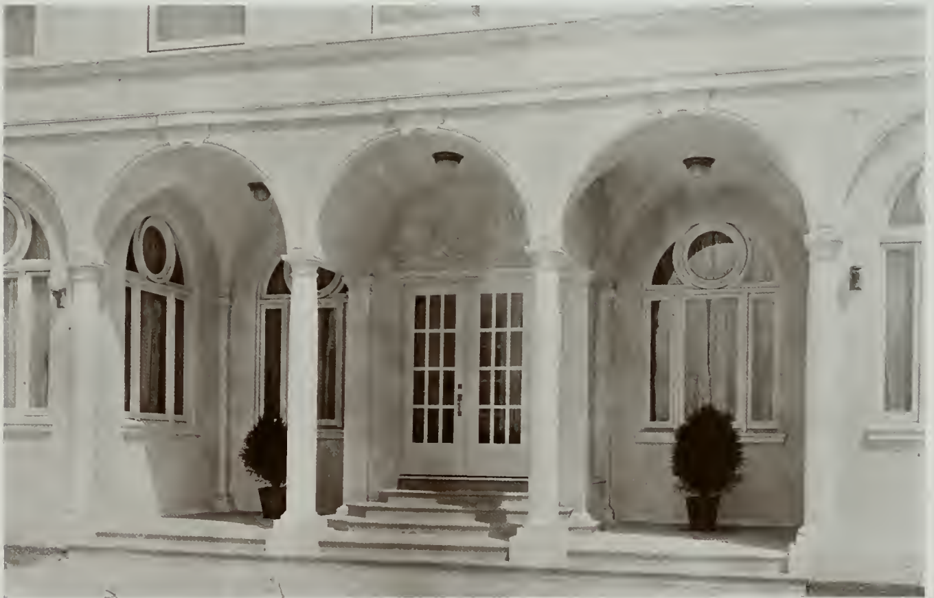
DETAIL OF ENTRANCE
