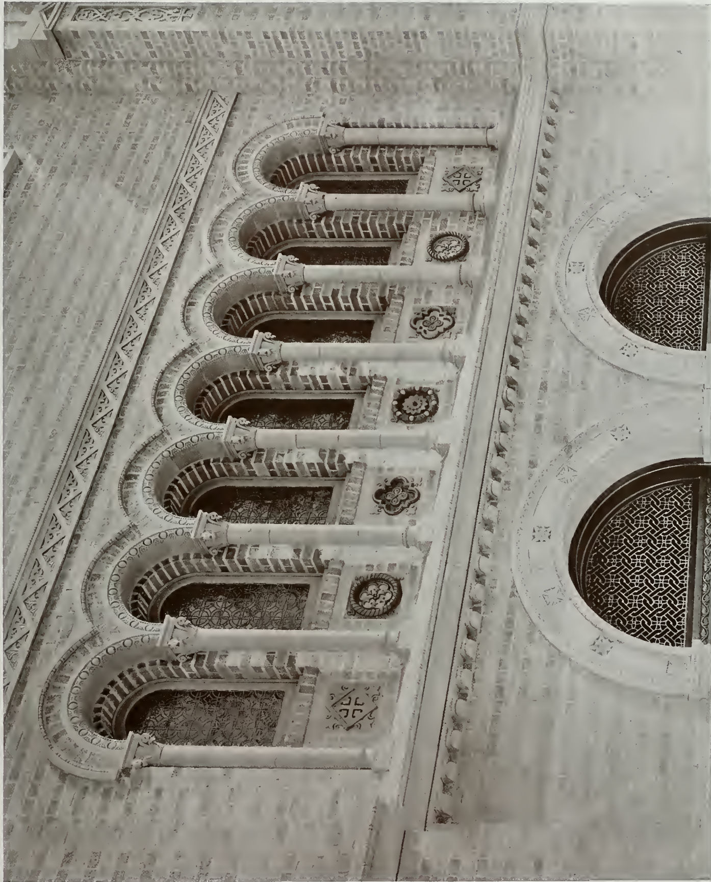
DETAIL WINDOWS OVER LOWER VESTIBULE ENTRANCE THIRD CHURCH OF CHRIST SCIENTIST, SAN FRANCISCO, CAL.
