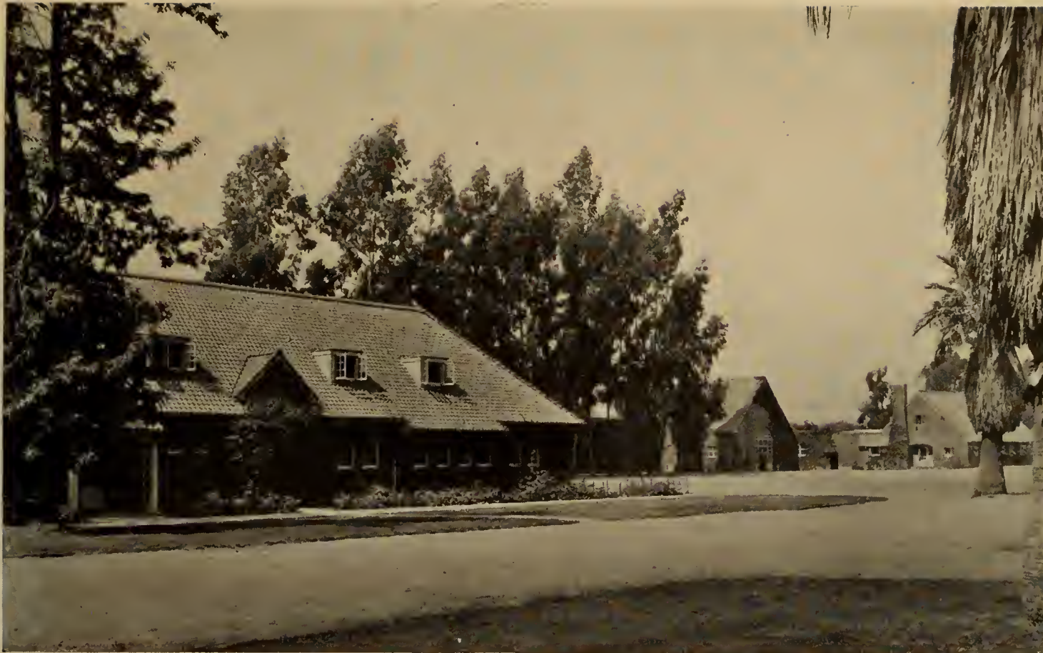
BOYS' COTTAGE, No. 11, WHITTIER STATE SCHOOL WHITTIER, CALIFORNIA GEORGE B. McDOUGALL, ARCHITECT
