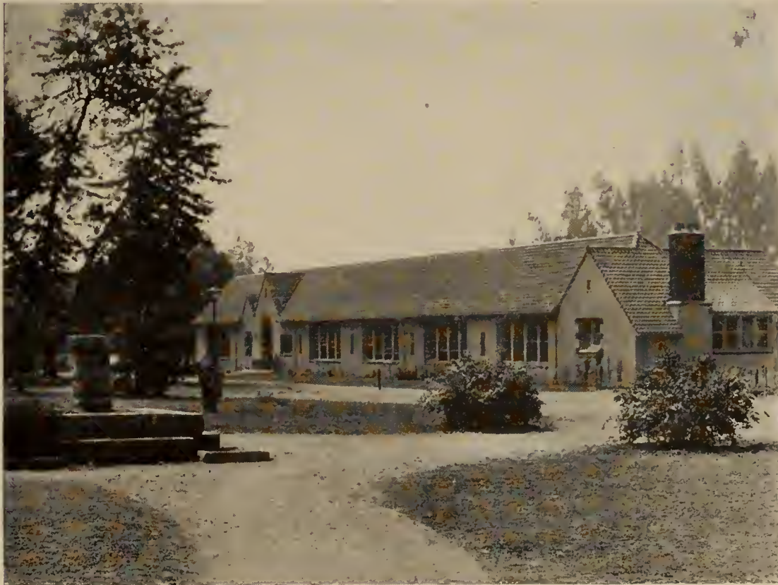
MAIN ELEVATION, SCHOOL BUILDING
