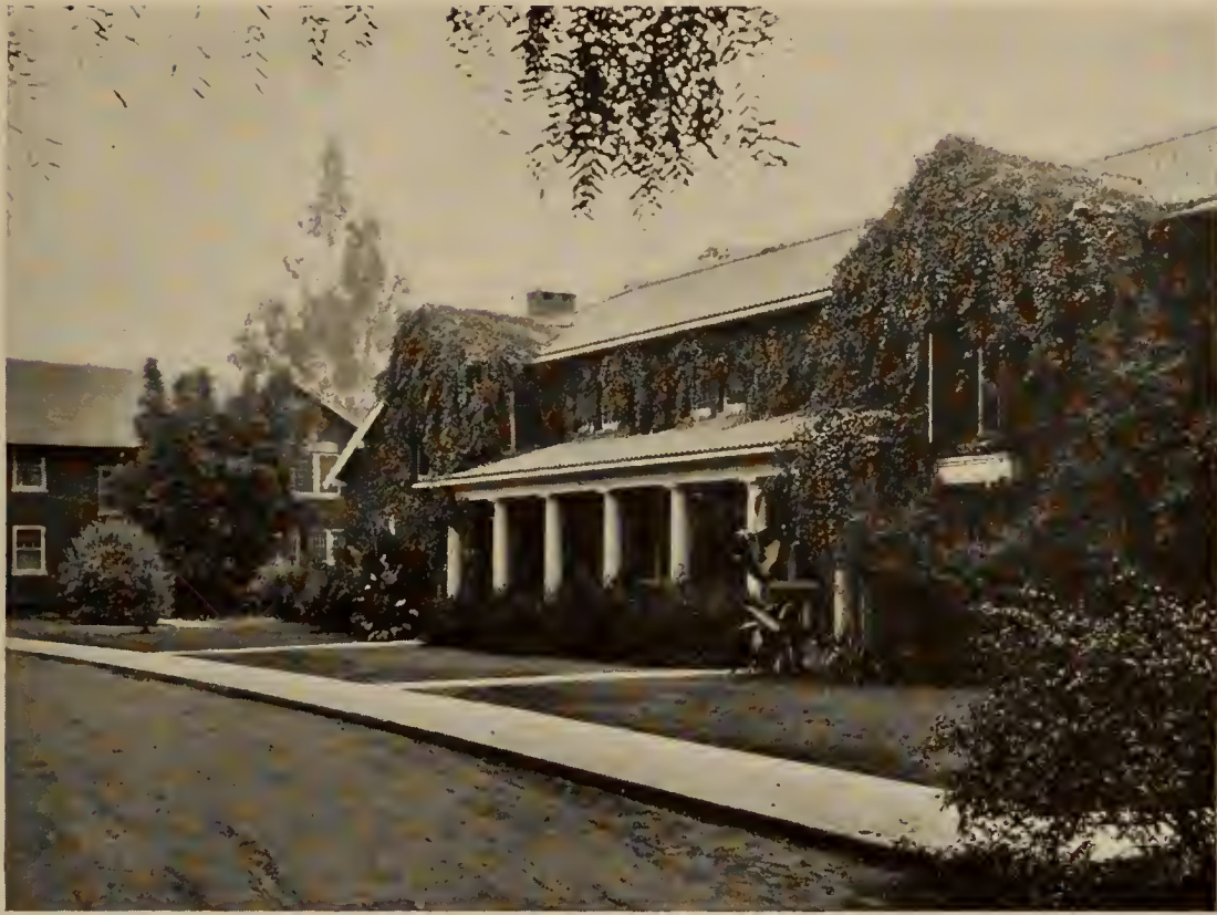
MAIN ELEVATION, HOSPITAL BUILDING
