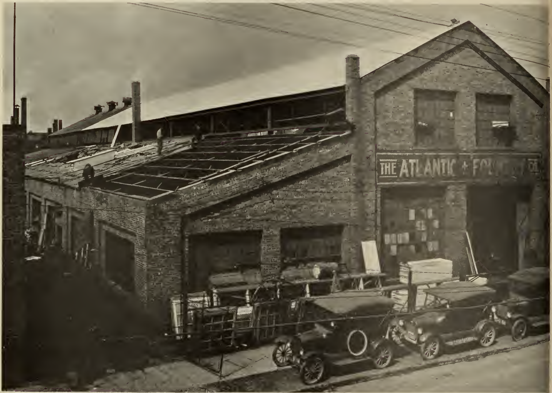
View of removal of Concrete Tile and application of
