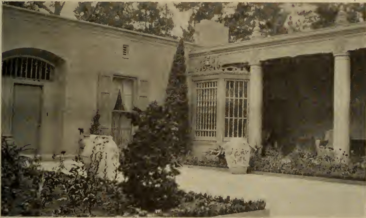
PATIO, COL. POOLE'S HOUSE, PEBBLE BEACH, CALIFORNIA. LEWIS P. HOBART, Architect.
