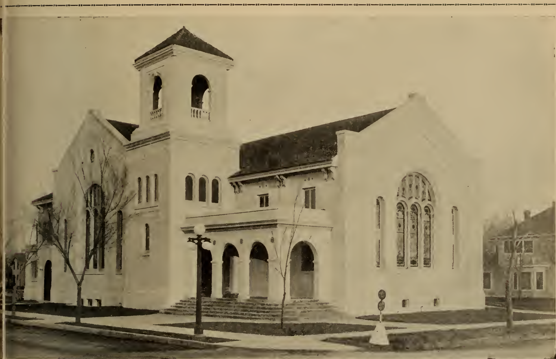
ROOFED WITH SIMONS LARGE SPANISH TILE.
