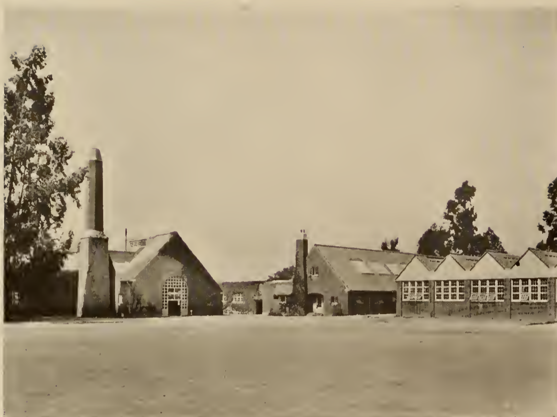
VIEW OF INDUSTRIAL COURT, SHOWING POWER HOUSE, LAUNDRY, BOILER AND PRINT SHOPS
