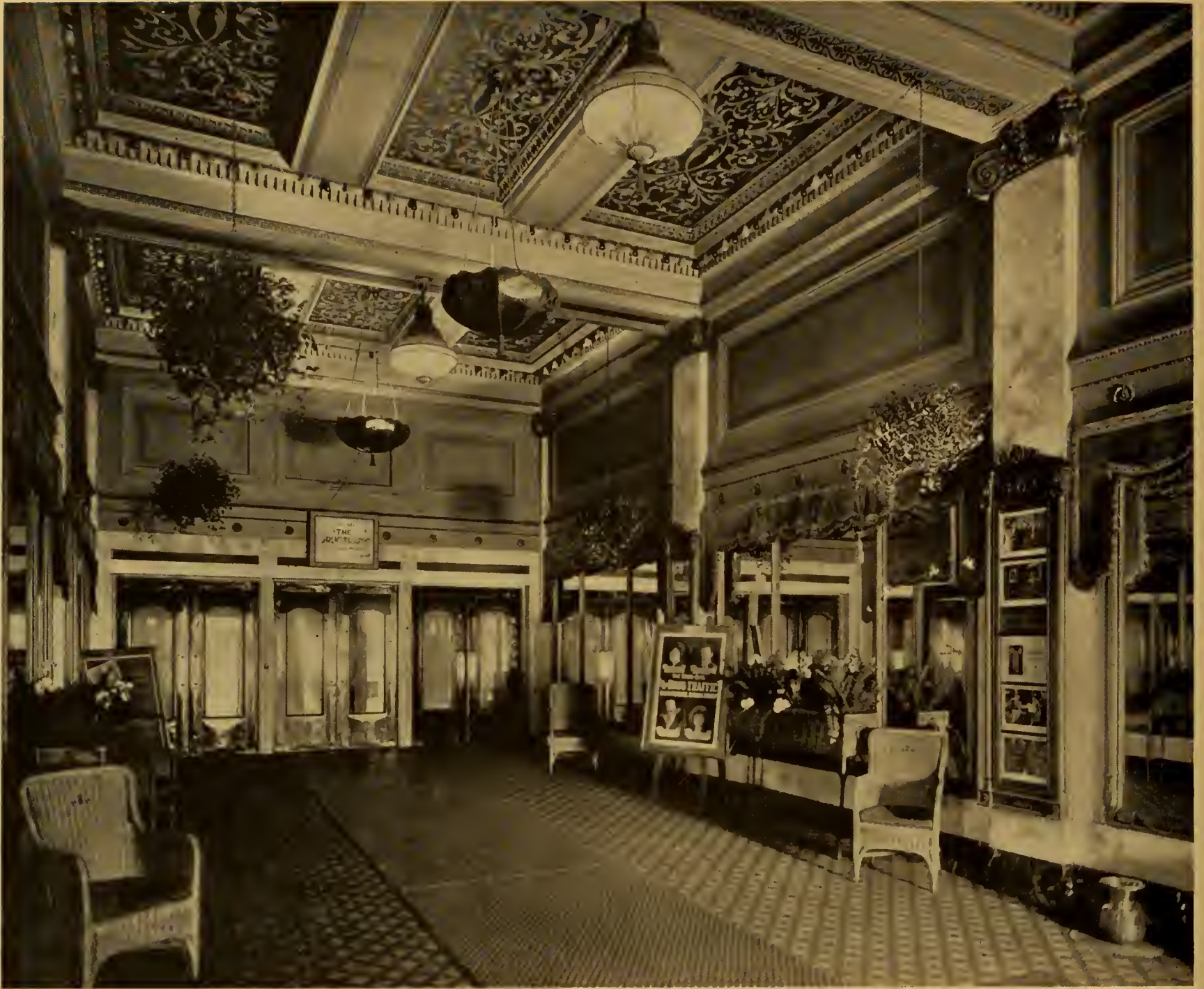
INTERIOR VIEW ENTRANCE LOBBY
