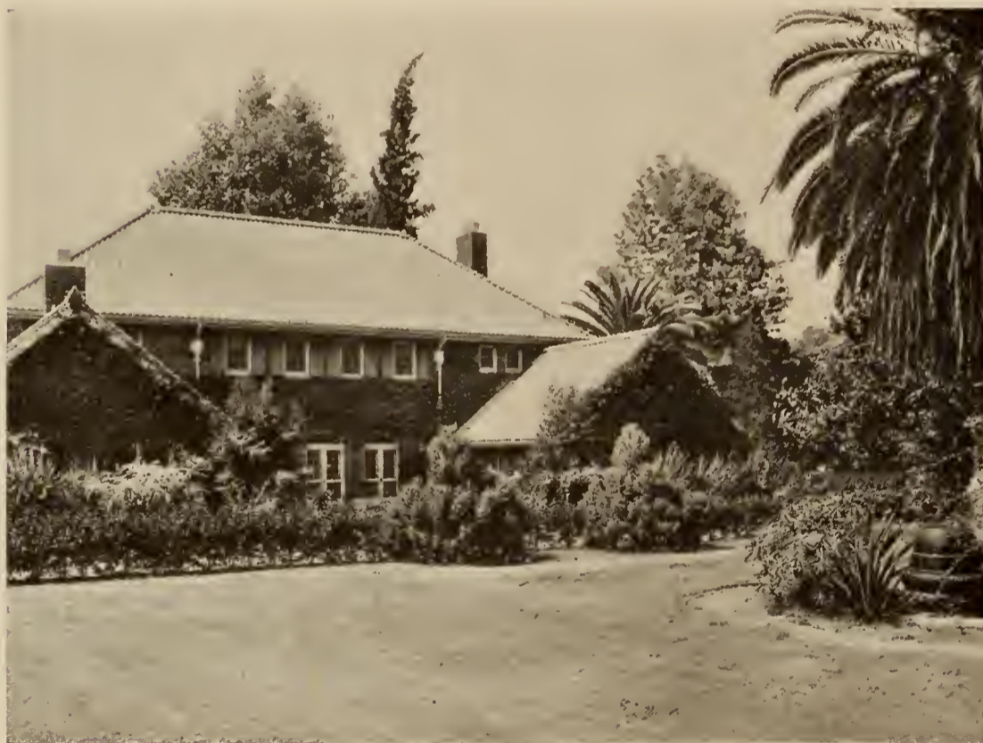
REAR OF BOYS COTTAGE No. 10
