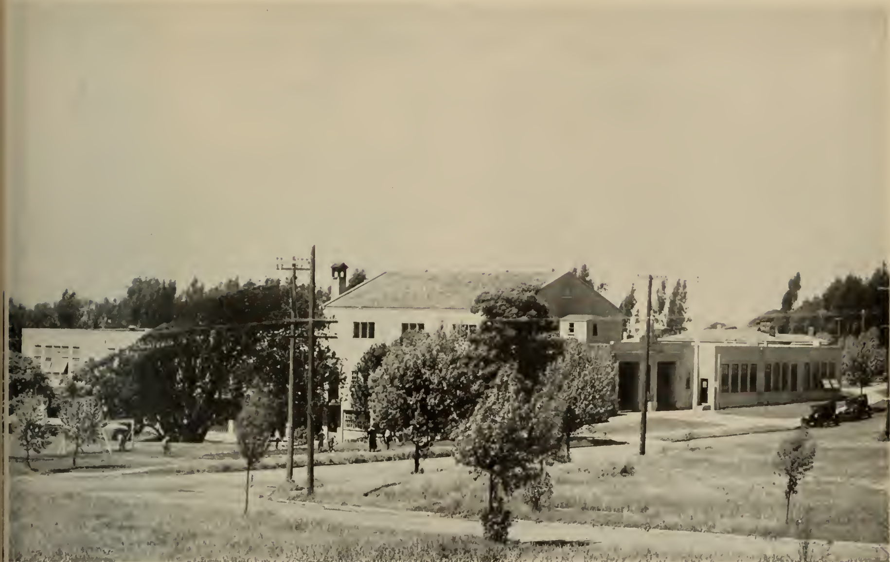
THOUSAND OAKS SCHOOL, BERKELEY, CALIFORNIA.
