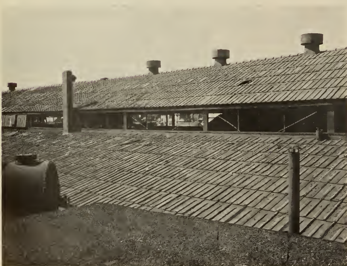
View before removal of Concrete Tile
