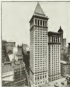
BANKERS TRUST COMPANY BUILDING. NEW YORK Marc Elditz & Sons, Contractors Trowbridge & Livingston, Architects
