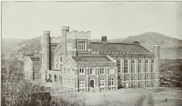
MACKY AUDITORIUM, UNIVERSITY OF COLORADO, BOULDER, COLORADO Gove & Walsh, Architects, Denver.
