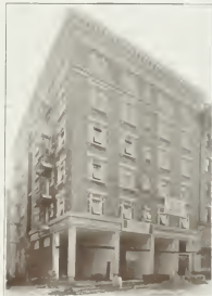
1077 L BUILDING 1077 L STREET - MICHIGAN STREET CORNER S. SCHNITZLER ARCHITECTS
