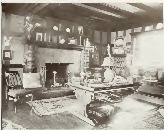
Living Room, Residence Mr. Edward Hobbes, Berkeley, Cal. Mr. Albert Fair, Architect, San Francisco, Cal.
