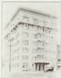
APPLEGATE HOUSE Made with N. Clark & Sons' Terra Cotta T. S. KILGUS ARCHITECT P. J. WALKER BUILDERS
