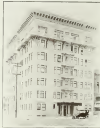
APARTMENT HOUSE Bush and Van Ness Avenue DUNN & KEARNS, ARCHITECTS R. W. MOLLEN, BUILDER
