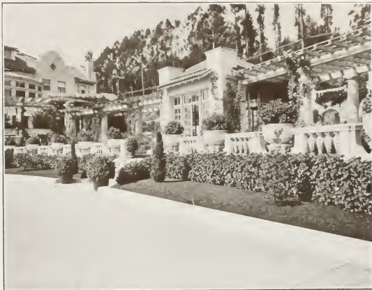
Garden Front, Residence H. H. Hart Oakland, Calif. C. W. Dickey, Architect Oakland, Calif.
