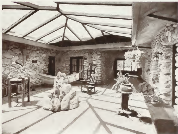
View in Court, Residence of Mr. Lee C. Pitzer, Pomona, Cal. Mr. Robert H. Orr, Architect, Los Angeles, Cal.
