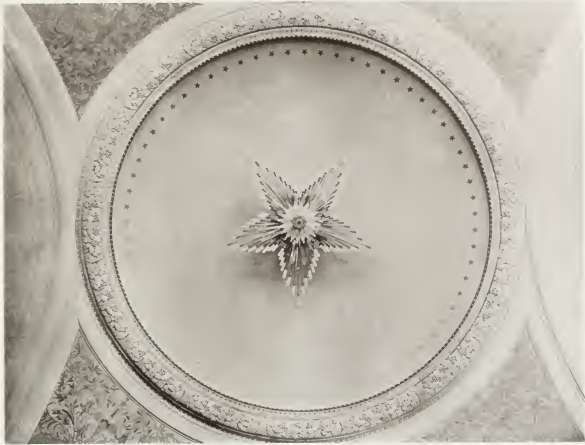
Ceiling of Eastern Star Lodge
