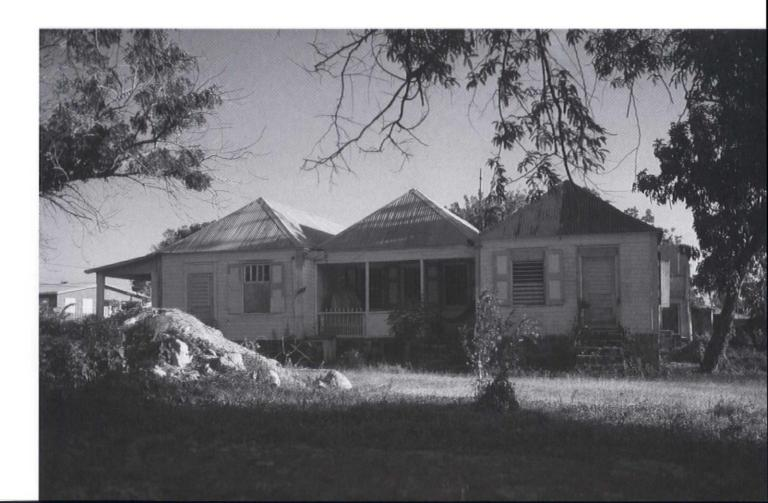
the common practice of recessing the hipped roof from the edge of exterior walls (rain water, gathered in a gutter atop the wall, is diverted to cisterns).<sup>12</sup>
