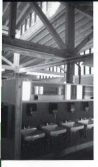
above: The Music Shed restroom building incorporates both ventilating clerestory awning windows and fixed clerestory glazing. Rafters and trusses are left exposed.
