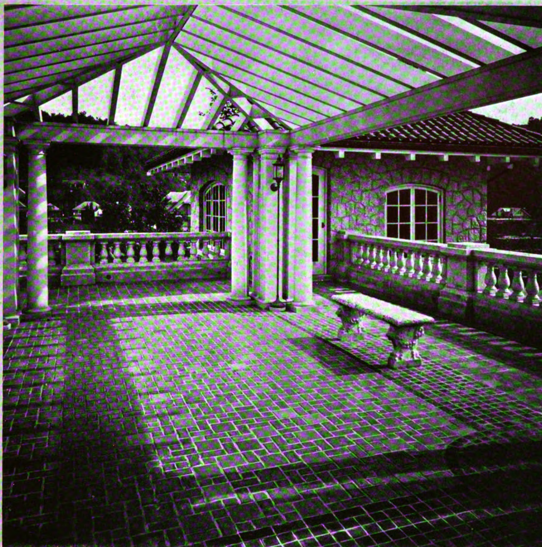
Roof Garden: House F. C. Pritchard, Huntington, W. Va. Floor of Copper Red Faience with border in colors JOSEPH HORNE Co., Designers
