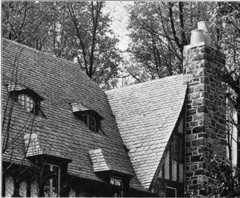
Residence, Glenwoolde, Long Island
