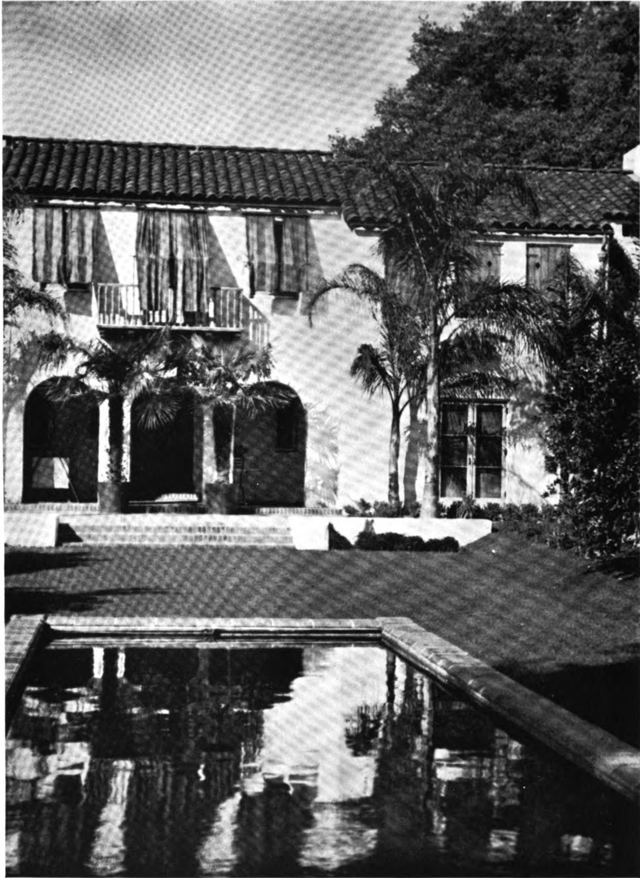
Johnson, Kaufmann & Coate, Los Angeles, Architects
