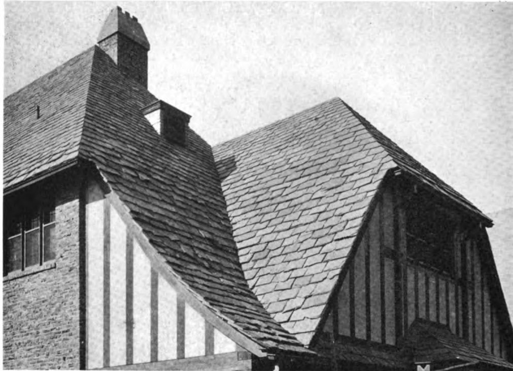
Raphael Hume, Architect
