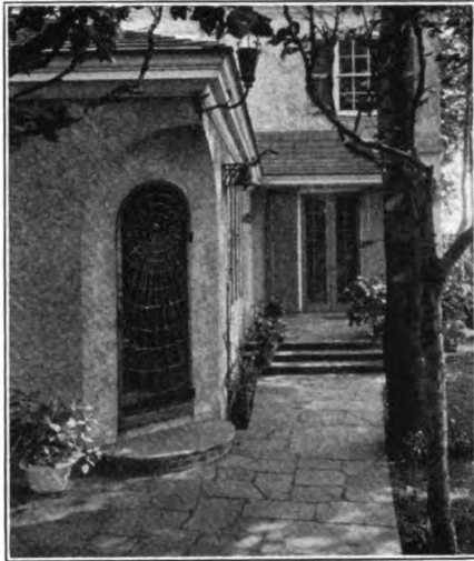
Terrace of Mrs. Meigs residence, Radnor, Pa. Mellor, Meigs & Howe, Architects
