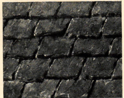
Detail of IMPERIAL Antique Shingle Tiles, showing how closely they approximate the roof of the centuries-old English cottage pictured above
