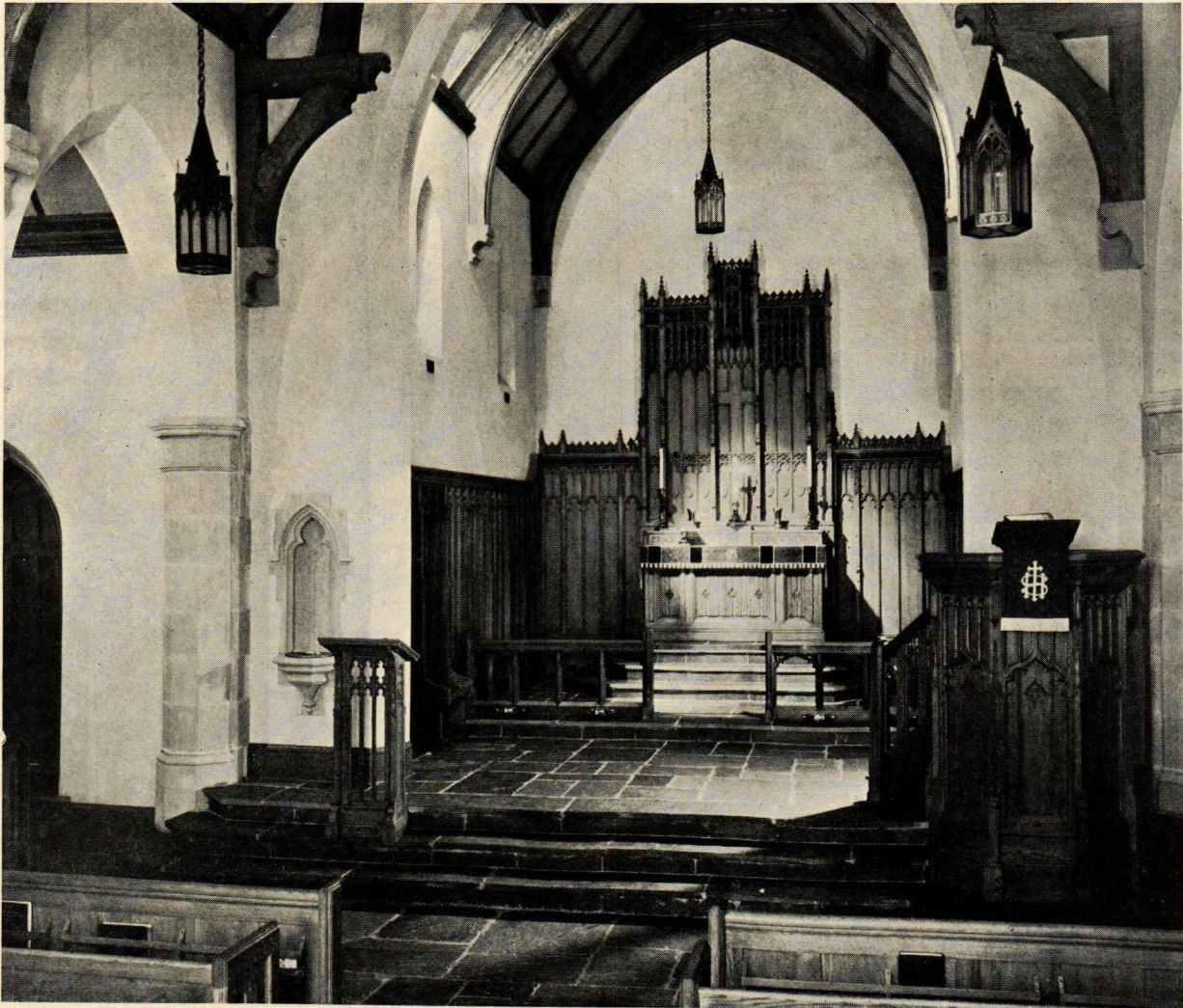
TRINITY EVANGELICAL LUTHERAN CHURCH, SCHENECTADY, N. Y. GEORGE W. CONABLE, ARCHITECT MADE AND ERECTED BY US
