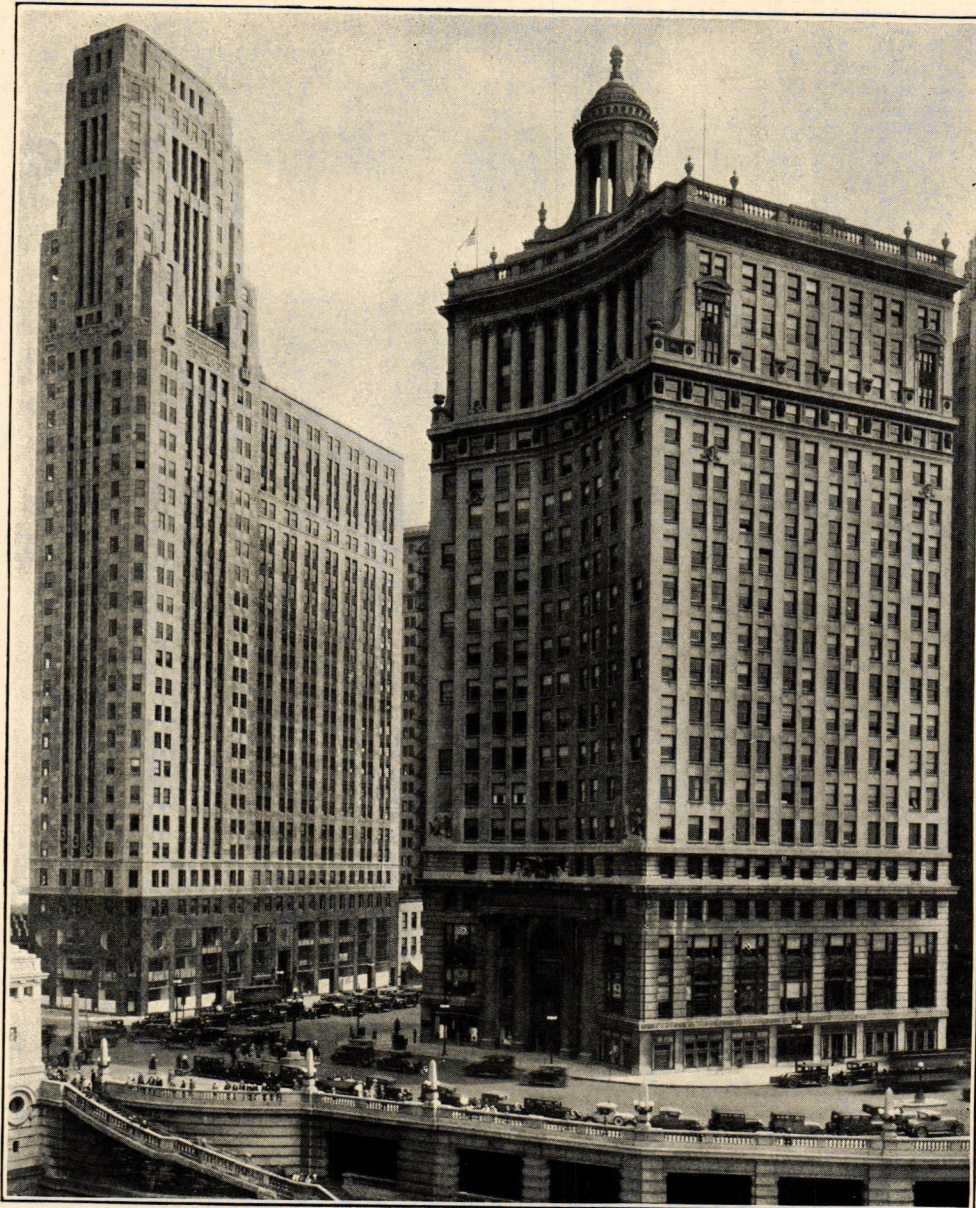
"333" N. Michigan Ave. Building, Chicago. Holabird & Root, Architects. Hegeman-Harris Co., Builders. Built of Shot-sawed Variegated Indiana Limestone. This photograph shows how Indiana Limestone predominates in Chicago's newer buildings.
