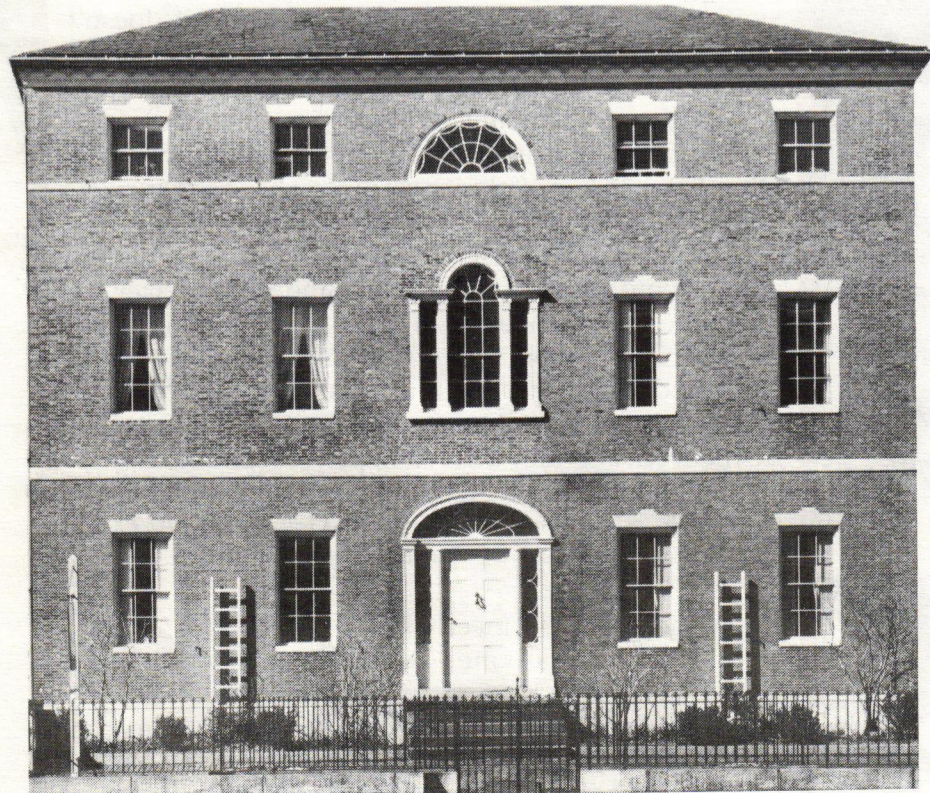
. . .While a mile away, a single elegantly detailed Palladian window fills its original role as an accent for a central entrance bay on this 1796 Federal house designed by Charles Bullfinch. (Photo: Society for Preservation of New England Antiquities.)
