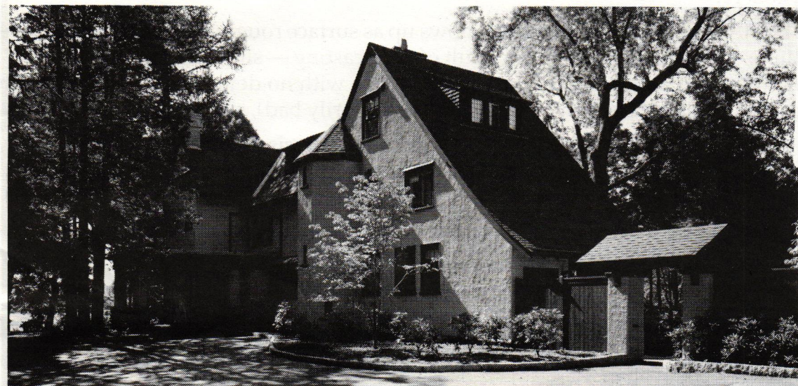
. . . and restoration of Fench House at Wellesley College . . . (Architects: Ann Beha, Marilyn Brockman, for Ann Beha Associates. Photo: Herb Engelsberg.)
