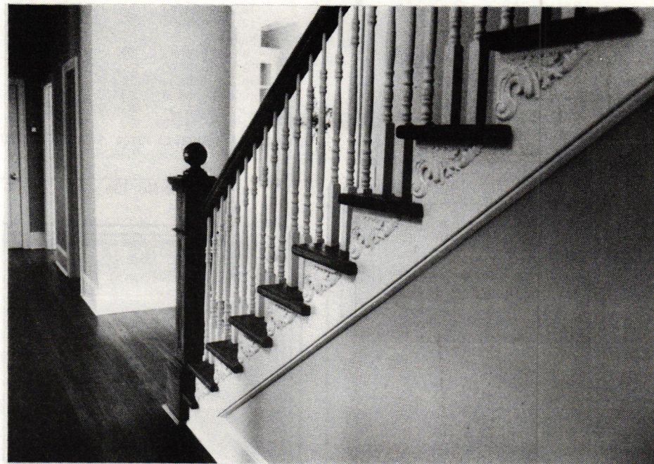
Locating architectural details, like the newel, balusters, and spandrel ornaments on this staircase, proved difficult for some of Bullock's customers. So she set up Specialty Building Supply to furnish historical millwork that builders can't find locally.
