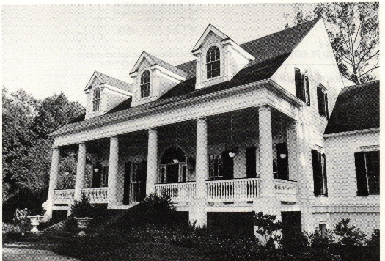
For her own family, Cecilia Bullock built this house in Jackson, Miss. — an adaptation of Historical Replications' Avondale Plantation plan. Built on a flood plain, the house was designed to handle a 1,000-yr. flood.
