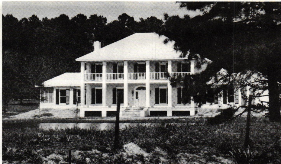
Cecilia Bullock has tapped into the architectural tradition of her native South, offering dozens of designs that are authentic renditions of antebellum houses.
