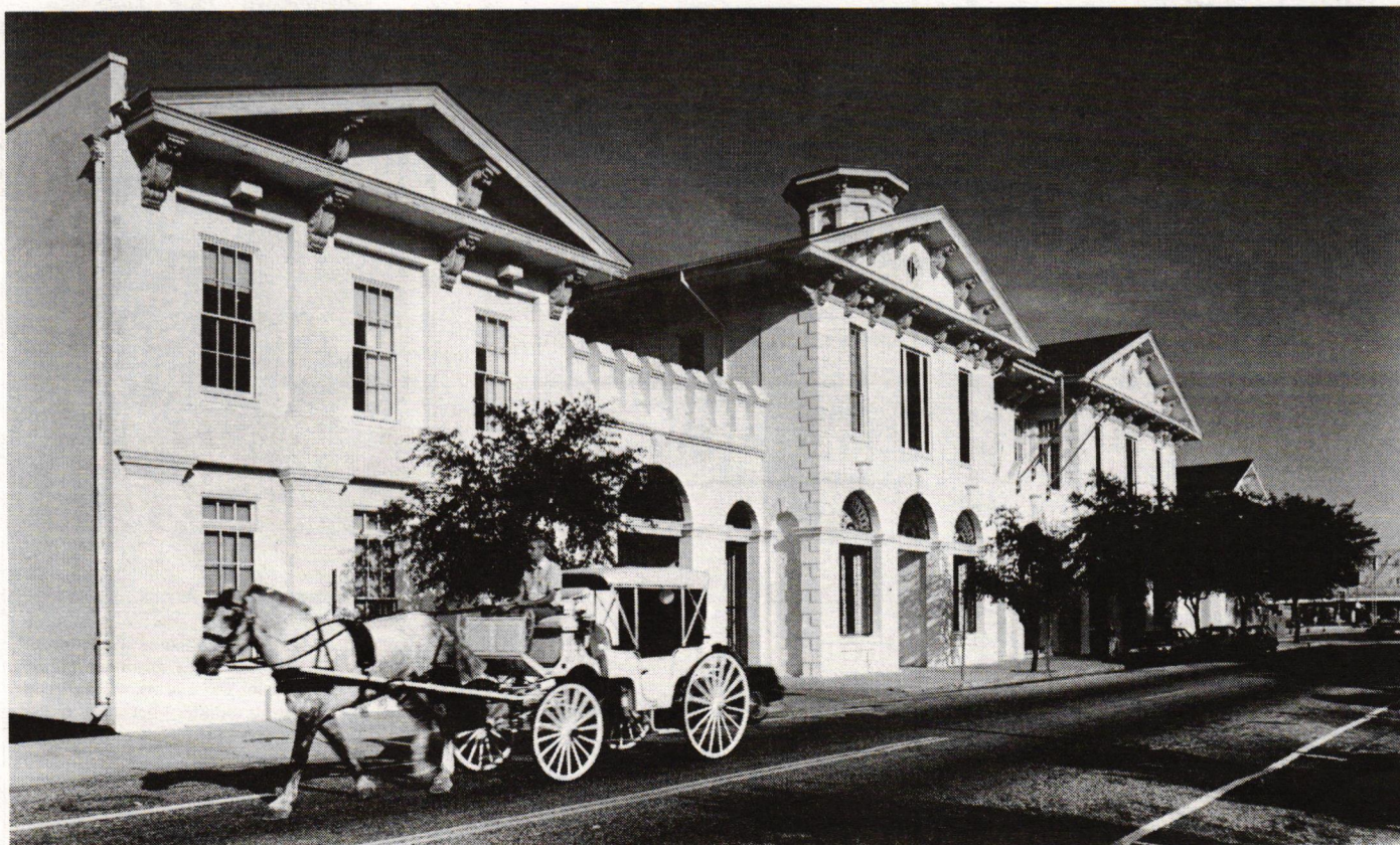
Mobile City Hall, built in 1857, was devastated by Hurricane Frederic. The Holmes firm did three complete sets of drawings for its repair: (1) Drawings for temporary repairs; (2) A full set of drawings for the insurance adjusters; and finally (3) A set of drawings for the restoration that, among other things, removed many decades of accretions.
