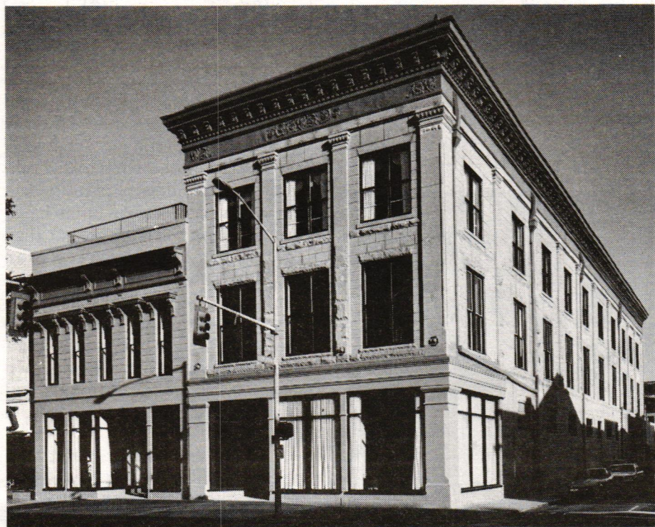
A Tax-Act rehabilitation in downtown Mobile converted an old Grant's department store to offices. Aluminum and enamel storefronts had to be removed from the facade; the Holmeses designed a new front similar to the original.
