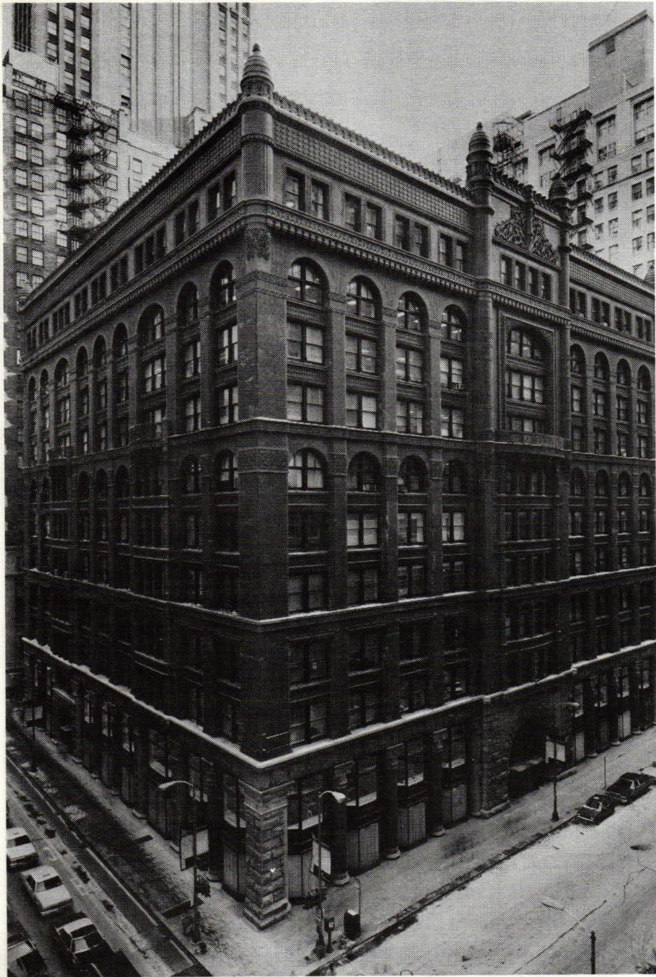
Burnham & Root designed the Rookery in 1888, Wright reworked its interior in 1904, and Hasbrouck restored it in 1990. Photo: Hedrich Blessing
