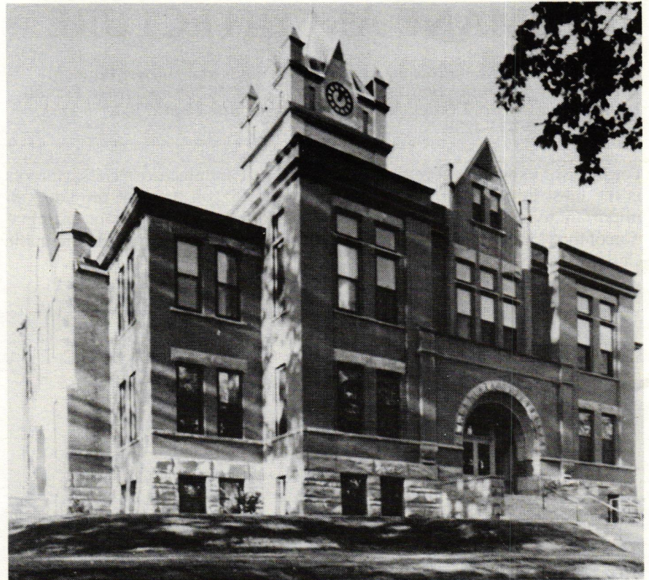
Hasbrouck met partner James Peterson when the two collaborated in 1981 on revamping the Grand Traverse County Courthouse in Traverse City, Michigan. Photo: Jack H. Murchie
