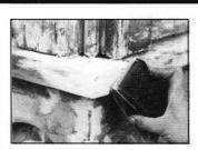
**LiquidWood** and **WoodEpox** give new life to severely rotted windowsills, sash, frames, shutters, columns, antiques, decorative wood elements. The Abatron system is especially valuable when original wood must be saved for historic reasons. **LiquidWood** consolidant reinfor-
