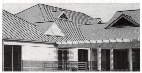
The high-seam profile design on this Tyler, Tex., golf resort roof incorporates an integral seam for panel engagement supplied by AEP-SPAN.
