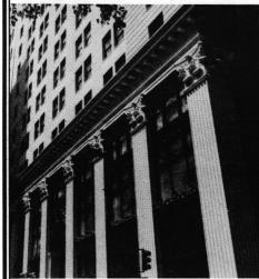
Restored facade of Widener Building. Capitals and horizontal ornamentation were made of fiberglass reinforced polyester resin in Polytek Rubber Molds.
