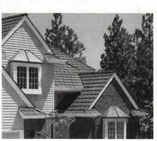
Wood-fiber cement shingles from AMERICAN CEMWOOD simulate the look of a wood roof and carry a Class A fire rating.
