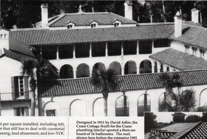
Crane Cottage (built for the Crane plumbing family) sported a then-unheard-of 16 bathrooms. The roof, shown here before the extensive 1992 renovation, is made from small tapered custom-manufactured Ludowici mission tiles.
