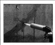
**ABOJET** structural crack-injection resins are proven to restore structural integrity to cracked load-bearing elements, such as foundations, abutments, swimming pools, concrete pipes, columns, and sculptures. **ABOJET** resin is injected into the crack, filling and welding it. **ABOJET** makes a permanent bond that is stronger
