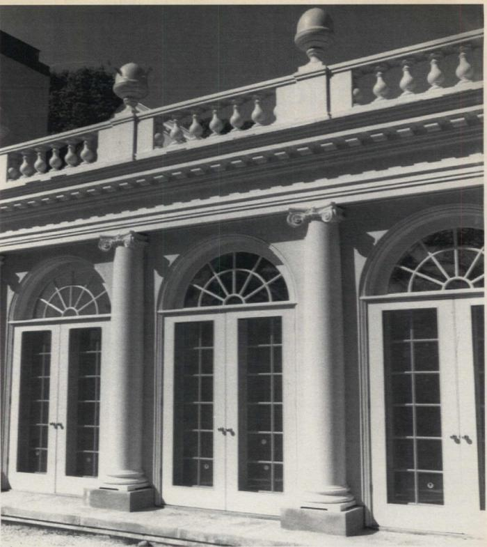
Balustrades are normally made "elbow height" — roughly three feet high, regardless of the scale of the building. For this Classical pavilion, however, architect Alvin Holm made the crowning balustrade only slightly higher than two feet. This has the effect of making the building seem larger than it actually is, lending a palatial quality to a house actually rather modest in size.
