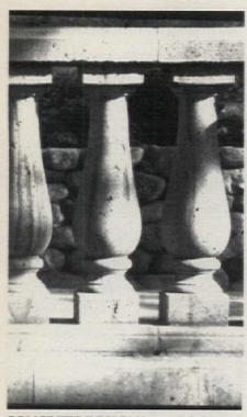
CONCRETE DESIGNS created this simulated Travertine cast-stone balustrade, along with columns, wall caps, and door and window surrounds for a residence in Southern California. All the elements were finished with an antiquing finish. Write in No. 5190
