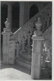
JONATHAN PETEFISH cast this staircase — treads, newels, flooring, baseboard, and coping — in a very dense hydraulic pozzolanic cement, for a custom indoor garden in Atlanta. Each step has five cast pieces on each side; they make up the tracery system and are bonded together with a structural epoxy. The inside of the handrails are hollowed, allowing for cable lighting to be installed behind each frond. Write in No. 8950
