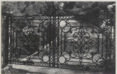
DESIGN ASSOCIATES supplied this forged-solid-steel lattice gate, incorporating details from the house into the design. The 16-ft.-wide, 5-1/2-ft.-high gates utilize FAAC hydraulic operators.
