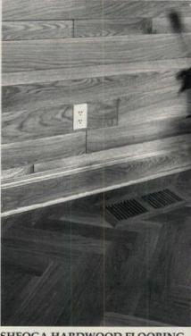
SHEOGA HARDWOOD FLOORING manufactures the 3-1/4-in.-face white oak herringbone flooring, white oak paneling, and flush-mount vent and frame, all shown here. Write in No. 1660
