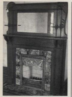
BUCKLEY RUMFORD rebuilt the inside of this Victorian-era gas-conversion fireplace in Columbus, Ohio. The original fireplace was coal, then it was converted to gas. To meet modern codes and keep the fireplace operable, they had BUCKLEY RUMFORD convert it to a Rumford fireplace. Write in No. 2590
