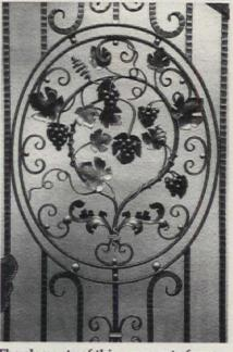
The elements of this grape gate from ARCHITECTURAL IRON DESIGNS include forged grape bunches, grape leaves, forged vine bars, and corkscrew twists. Write in No. 7950
