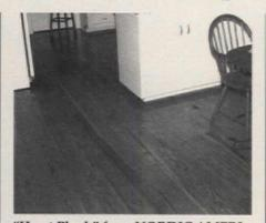
"Heart Plank" from NORDIC AMERI-CAN CORP. is a salvaged antique heart pine that is kiln-dried, milled, and then laminated into a strong, fiveply laminated floor that can be installed directly onto a variety of subfloors.
