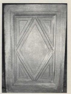
This approximately 3-ft.-sq. precast concrete block was replicated by KEY CAST STONE after an existing one, to match a balustrade system for a church in Astoria, Queens. Write in No. 4700
