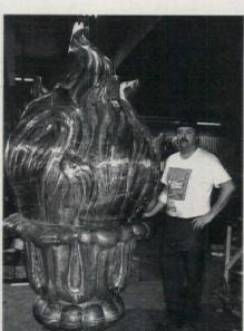
HEATHER & LITTLE, LTD., recently completed the replication of the Flame of Knowledge finial that perches on the main dome of the Library of Congress in Washington, D.C. The finial stands close to 16 ft. in height. All pieces were hand-formed, riveted, and soldered together. Write in No. 2470
