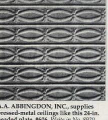
A.A. ABBINGDON, INC., supplies pressed-metal ceilings like this 24-in. beaded plate, #606. Write in No. 8920
