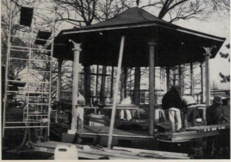
The gazebo in Trophy Park at the Norfolk Naval Yard in Virginia was an excellent project for the carpenters in training. The 1/8-in. accumulation of paint also served as training ground for an extensive lesson in lead-based-paint removal.
