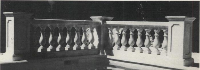
ECOPIC baluster molds, made of talc-reinforced polyethlene, can be used to create interior and exterior balusters in such materials as plaster and concrete. This Mediterranean poolside has balusters made from one of their molds. Write in No. 7090
