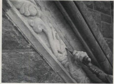
Jahn M70 limestone-sandstone mortar from CATHEDRAL STONE PRODUCTS can be used for minor patching or total reconstruction of ornamental stones. Here, the material is being carved in place during the ornamental-sandstone repairs at St. Patricks Church in Washington, D.C. Write in No. 9580
