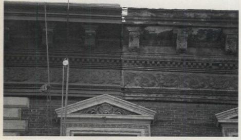
ARCHITECTURAL FIBERGLASS CORP. created an FRP replication of the sheet-metal cornice of this apartment building on St. Nicholas Ave. in New York City. The cornice is 60 in. high with a 36-in. projection; the panels measure about 5 ft. 9 in. long. The photo shows the cornice prior to repainting. Write in No. 6400
