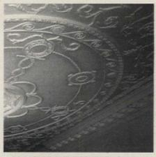
LUCZAK BROTHERS, INC., designed, fabricated, and installed this 20-ft.-x-30-ft. suspended plaster ceiling with applied moldings and cornice in a Chicago residence. Write in No. 1035
