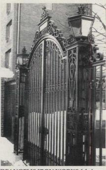
DEANGELIS IRON WORKS fabricated and installed a new ornamental fence and gate around the only unfenced area in historic Harvard Yard. The project involved precise duplication of the existing fence, which was installed in the 1800s. Gate scrolls were hand-forged, and new castings were made from molds of existing components. Write in No. 1023
