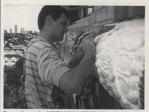
Here, a craftsperson from MOLDMAKING & DESIGN, INC., working nine stories up, removes a silicone mold taken from a terra-cotta ribbon ornament. The company provide fabrication and prototyping in addition to moldmaking, casting, and other restoration services. *Write in No.* 7270
