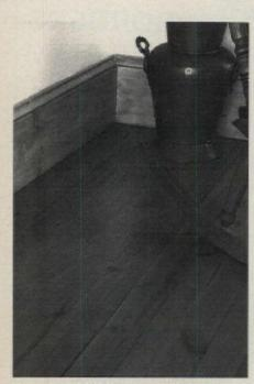
Here, CARLISLE old-growth Eastern white pine in random widths up to 20 in. wide was finished with a stain and a high-resin tung-oil finish, and installed using antique cut nails. Flooring is available in tongue-and-groove, ship-lap, or square-edge. Write in No. 5580
