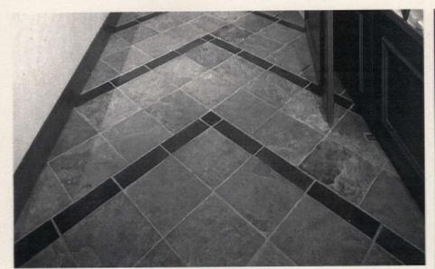
The Vivande Ristorante in San Francisco used ECHEGUREN SLATE as its flooring material; China lotus tiles measuring 12 x 12 in. and China black tiles measuring 12 x 3 in. cover the floor. Write in No. 7220
