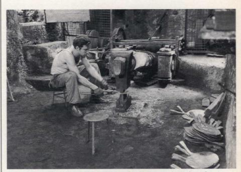
Here, John Crawford, during his apprenticeship in Tuscany (c.1979), works at a water-powered trip-hammer making "testi" (lower righthand corner). These griddles, used for roasting chestnuts, are made by first flattening out the paddle, leaving a tab, which is later drawn out into a handle.
