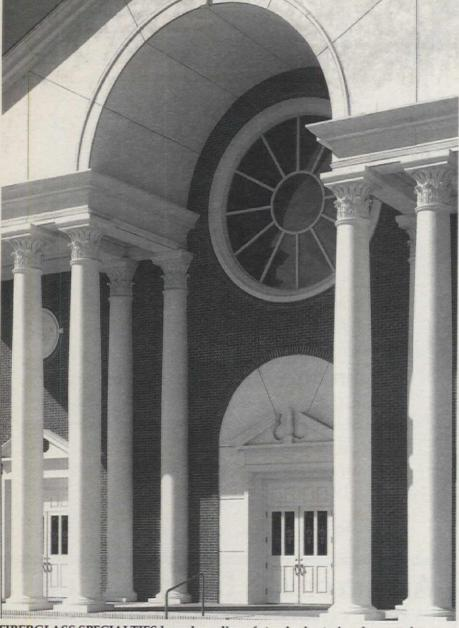
FIBERGLASS SPECIALTIES has a large line of standard exterior elements for churches and can also create custom-designed elements. Here, they supplied custom fiberglass columns, capitals, cornice, window and door surrounds, and door pediments. Write in No. 7310
