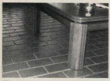
This 4-x-8-in. runningbond-brick pattern was created with ARTCRETE Faux Brick, using poured-in-place stenciled concrete, paper stencils, and a dry-shake color hardener. Write in No. 2140
