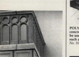
CALIFORNIA PRECAST STONE MFG. produced this unique balustrade assembly designed by a San Diego architect for an Italianate-style home. The finished product was a high-density casting with an etched finish resembling weathered limestone. Write in No. 8100
