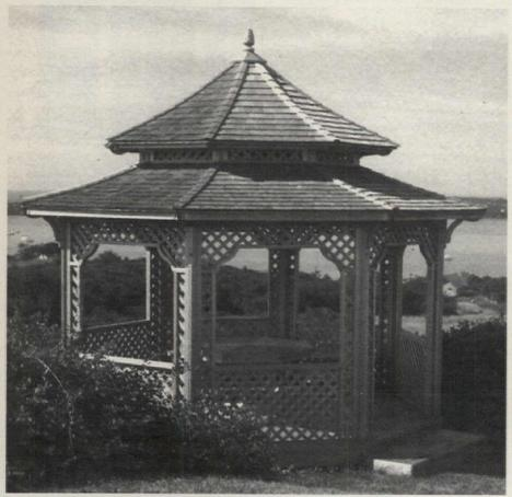
DALTON PAVILIONS' 15-ft. Victorian pagoda, shown here along Montauk Point in Long Island, N.Y., is fabricated from Western red cedar and uses stainless-steel fasteners. Write in No. 330
