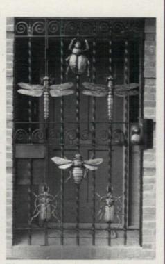
Dimensional beetles, dragonflies, and a bumblebee all swarm on this fantasy gate, an original design forged by PHILLIPS METALWORK for a residential client. The pickets, scrolls, and insects are all forged; the two bugs on the left are hinged with the gate.
