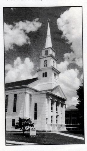
Built in 1834, the historic Congregational Church in Westborough was thoroughly renovated in the early 1990's. Fiberglass Specialties was chosen to fabricate the spire, top cupola, and eight urns. The shingle effect on the spire and the simulated wood siding of the cupola are in fact molded into the fiberglass laminate. And since the white color is an integral part of the laminate, eliminating the need for scraping and repainting, the church will save on maintenance costs in the future.
