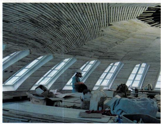
Above: The architects specified historic materials for the 77-ft.-dia. main dome – wood lath and lime plaster – to follow Latrobe's intent and because they realized that these materials had the flexibility needed to accommodate the movement of the outer wooden dome. Photo: courtesy of the Baltimore Basilica
