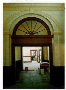
Architectural Components built the custom lunette, door frames, casing, chair rail and wainscoting to match the existing elements of this building.
