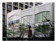
The glass fiber reinforced concrete (GFRC) used to re-clad this building on State Street in Chicago, IL, was acquired from Ball Consulting.
