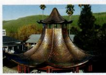
Vulcan Supply custom fabricated the shingles for this copper pagoda in its Vermont shop before completing the installation on site.
