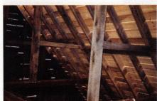
This timber-frame roof of this 60-ft. barn was replaced by Colonial Restorations using gin poles instead of a crane.
