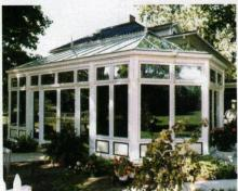
This conservatory by Glass House features custom details such as molding, gutters, downspouts, cresting and finials, leaded glass, French doors, interior ornamental eave bracketry and tension rods.
