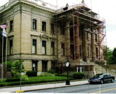
Above: Heavy-loading scaffolding was erected around the front entrance of the Marion County Courthouse while its cast-iron elements were repaired, cleaned
