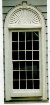
This reproduction 12/12 window with fan was fabricated by Architectural Components.
