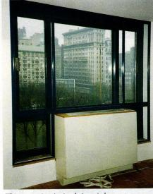
This custom interior insulating window system was fabricated by Cityproof.
