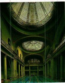
The grand art-glass domes of the natatorium at the Olympic Club in San Francisco were restored and engineered with a proprietary seismic system to protect it from earthquakes by Reflection Studios.
