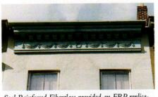
Seal Reinforced Fiberglass provided an FRP replication of the original metal cornice for this New York City building.
