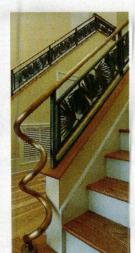
Robinson Iron designed and fabricated this elegant stair railing.
