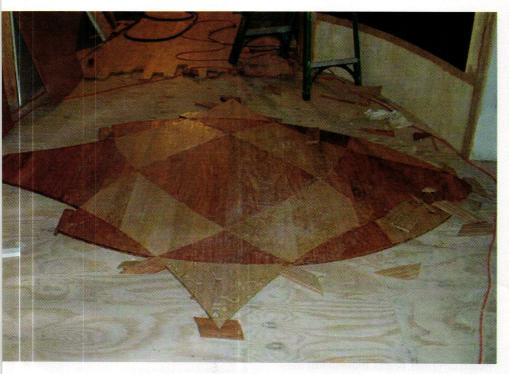
Above: Each section of the mosaic was made of multiple pieces of 3-in.-wide flooring and each was laid down like flooring, using adhesive and then nailed in place. Because 3/4-in. wood was used for the project, it will require very little maintenance.
