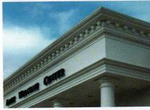
This cornice was built using pre-finished architectural urethane multi-profile moldings supplied by Melton Classics.
