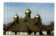
Five onion-style golden domes were custom manufactured and installed by Architectural Fiberglass on the Holy Trinity Church in Parma, OH; one measures 18x32 ft. and the other four are 15x26 ft.
