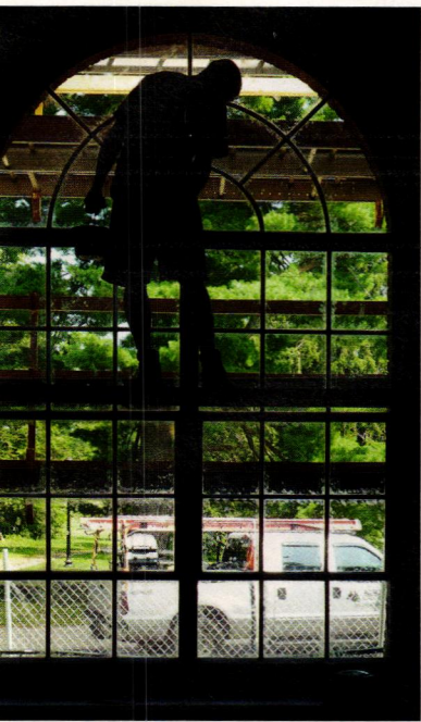
A Seekircher worker paints one of the windows at Ely Hall.
