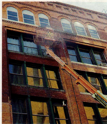
ArmaKleen manufactures Armex blast media, a baking-soda-based abrasive for gently cleaning brick and other substrates.
