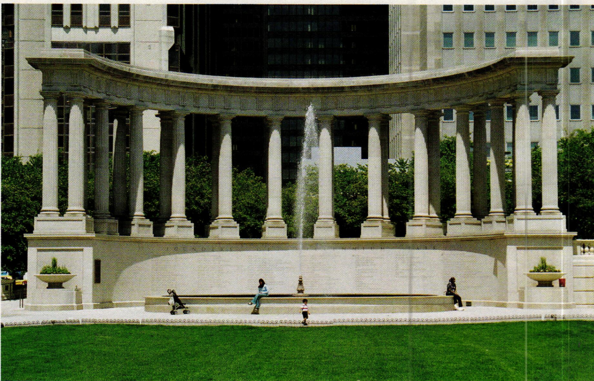
Bybee cut and carved the new peristyle in Indiana limestone for Chicago's Millennium Park. It includes 24 paired, fluted, 40-ft. tall Doric columns. Photo: Bybee Stone Co.
