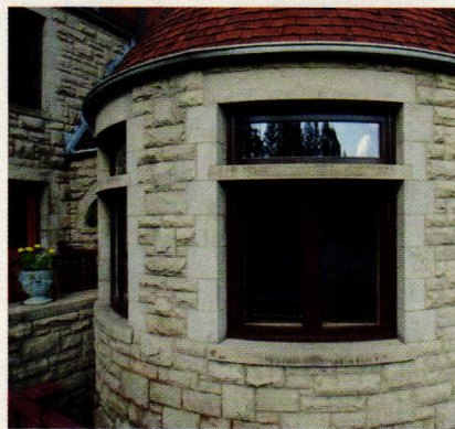
HeartWood supplied the replacement windows for this 100-year-old cemetery gatehouse in Rochester, NY; they are made of quarter-sawn white oak and bent glass.
