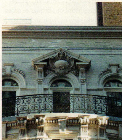
Architectural Fiberglass Corp. created the cornice and other decorative ornament for this building.
