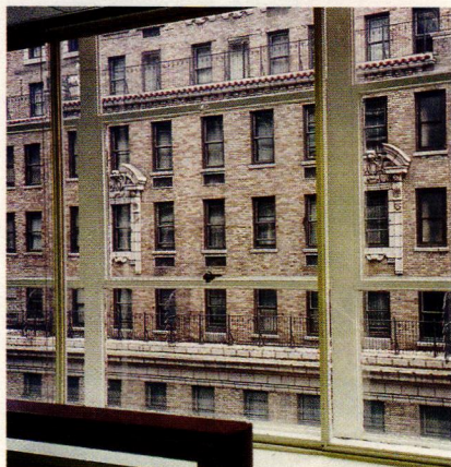
Interior storm windows from Cityproof windows are designed to reduce noise infiltration.
