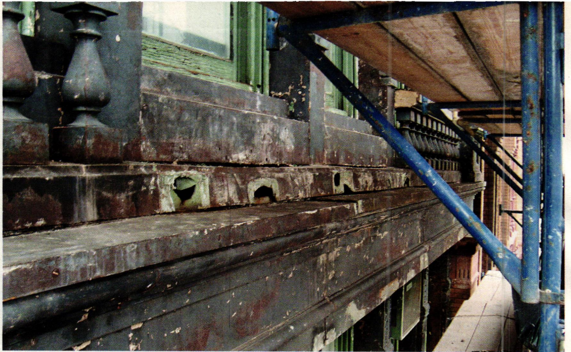
Middle: The sheet-metal sections on the upper floors required repairs to rust swaths, dents and punctures. Photo: Joe Polowczuk
