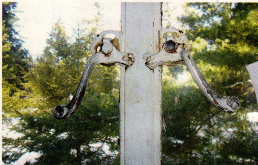
Over the years, the steel windows at Vassar had become encrusted with paint and were inoperable (left). After restoration (above), the windows were as good as new, providing light to classrooms and art studio. All photos: courtesy of Seekircher Steel Window Repair unless otherwise noted.
