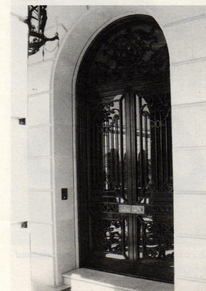
This 11-ft. custom bronze door was manufactured by Historical Arts & Casting with a patina formulated to age gracefully in any climate.
