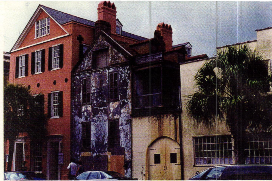
Before restoration, #97, like #93, was a ruin.
