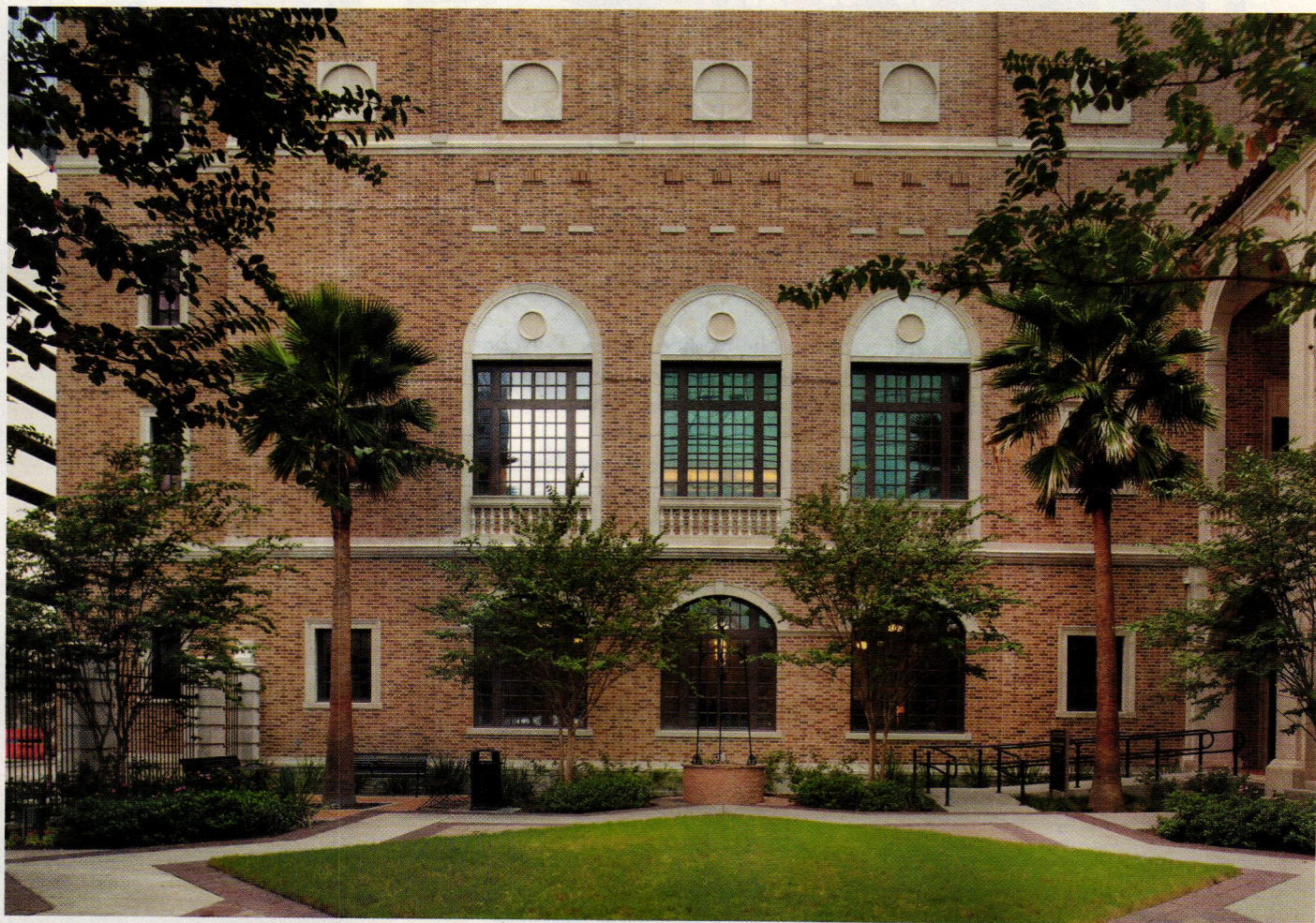
The exterior of the new addition was designed with simple details to appear as close “first cousins” of the existing building; the cast-stone arched loggia extends from the addition and frames an outdoor reading garden.
