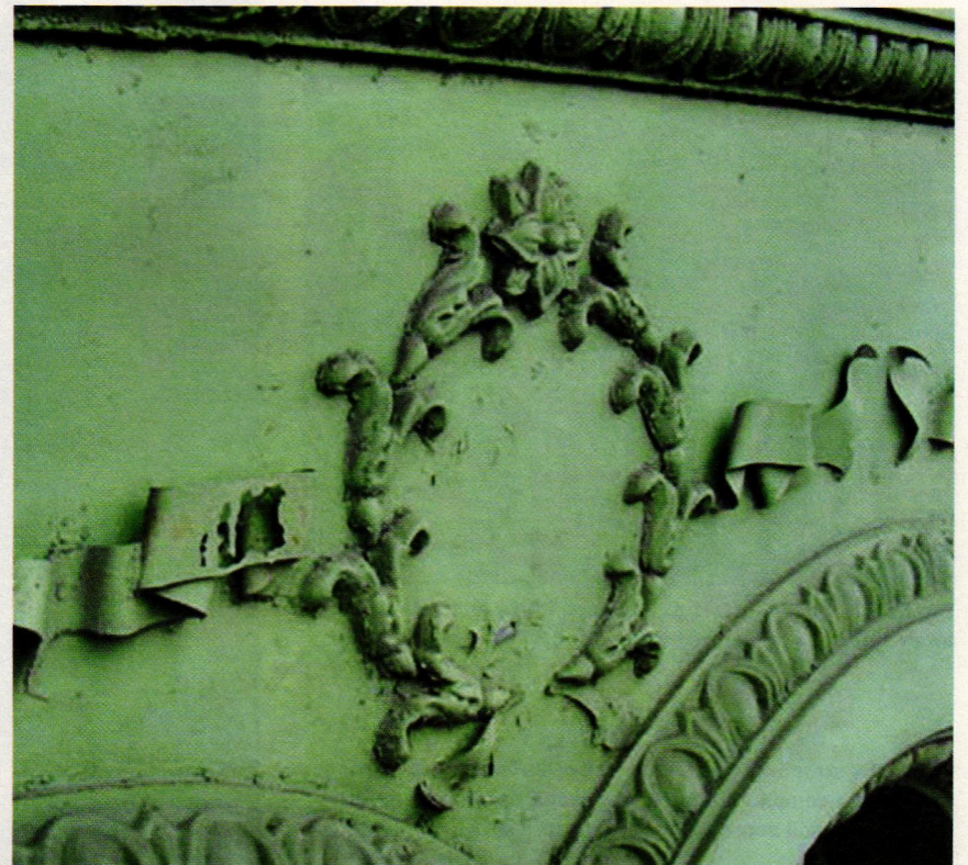
Below: The delicate ornament was literally eroding away. Photo: Joe Polowczuk
