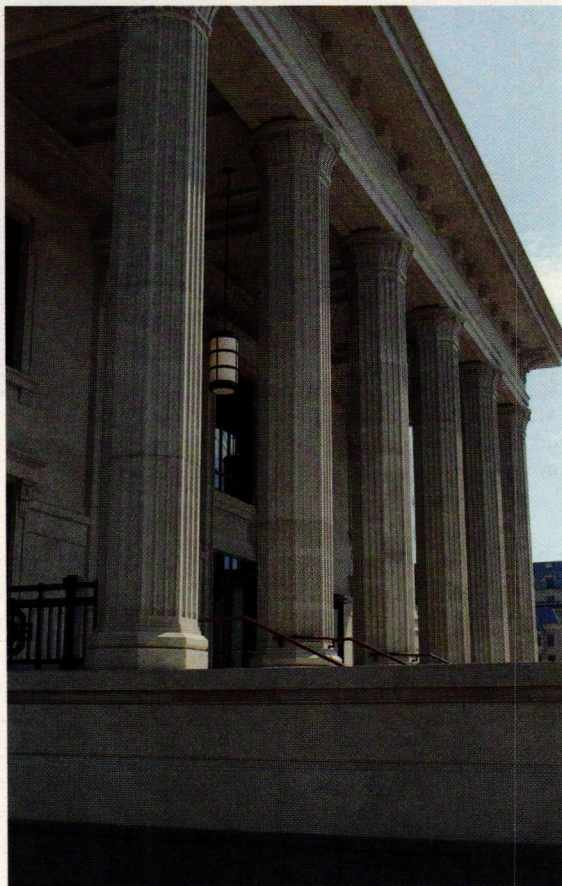
Bybee fabricated the columns for the Palladium at The Center for the Performing Arts, Carmel, IN. Photo: Bybee
