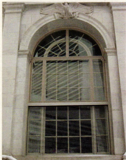
Allied Window supplied the Protective Allied One Lite (PAOL) exterior removeable storm windows for the Byron White U.S. Courthouse in Denver, CO.
