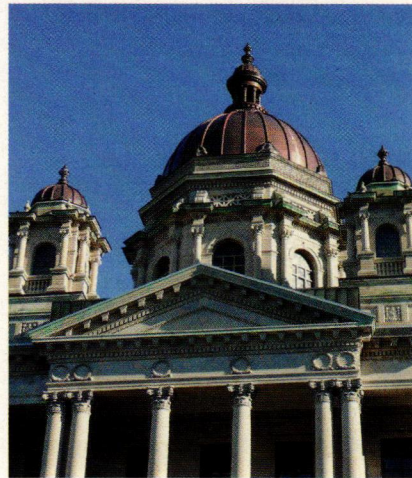
These domes for the Onondaga County Courthouse, NY, were fabricated by Heather & Little.
