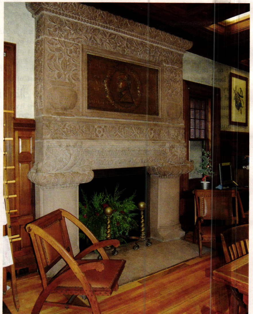
Now cleaned and restored, the mantel that was designed by Stanford White and carved by Augustus Saint-Gaudens is once again the focal point of the smaller reading room known as the mantel room.
