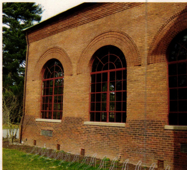
The largest windows at Vassar's Ely Hall are 7x11 ft. All are now restored. Photo: Andy Wilson, CVM
