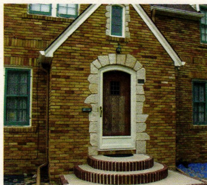
Arch Angle provided the storm windows and doors for this building.
