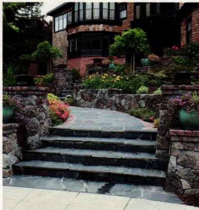
Reclaimed clinker bricks supplied by Gavin Historical Bricks were used to create these steps and walkway.
