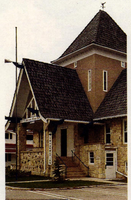
Vande Hey Raleigh supplied the charcoal-gray weather #2 black slate replica for the roof of this village hall in Ephraim, WI.
