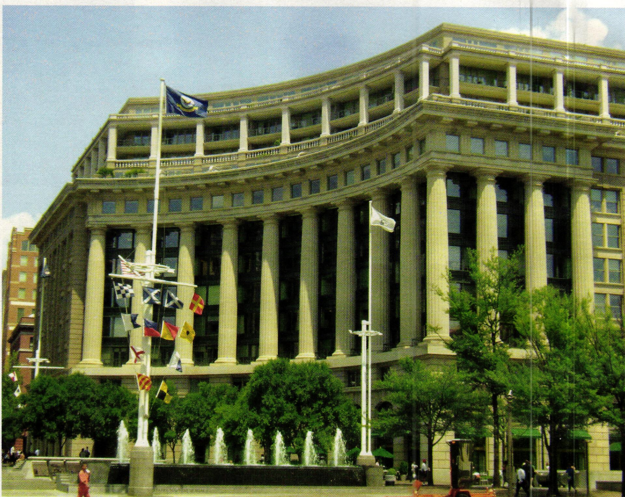
Market Square in Washington, DC, consists of two buildings with columns in a semi-circle around the Navy Memorial. Bybee Stone Co. fabricated 26 6-ft.-dia., 55-ft. tall, fluted, solid-limestone columns, complete with capitals and bases, for the project. Photo: Bybee Stone Co.
