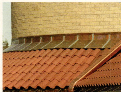
The roof tile for the restoration of St. Patrick's Catholic Church in Waukon, WI, features Ludowici's Spanish Tile in clay red.
