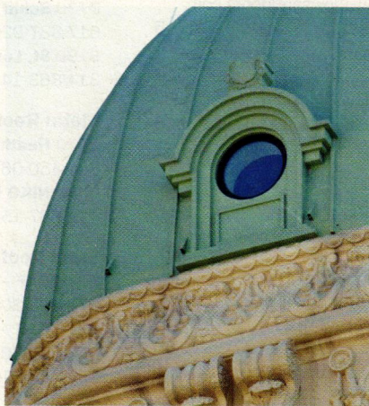
Gotham Metalworks fabricated this precision plasma cut replication domed roof for a NYC landmarked building.
