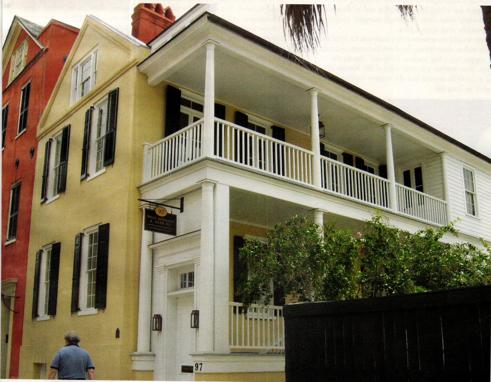
The residence at #97 Broad Street is typical of the historic housing stock in Charleston, with the narrow end facing the street. A double-height side porch, known as a ‘piazza’ in Charleston, faces south or west to catch the prevailing breezes.
