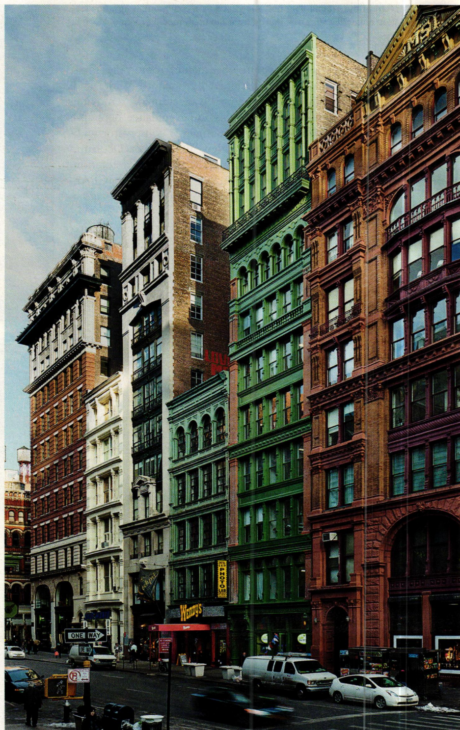
Similar adventurous experiments in lacy cast-iron façades, the precursors of modern curtain walls, surround the ten-story shaft of 648 Broadway. Photo: Jack Kucy
