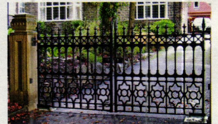
This iron gate for a 12-ft. opening was cast in one piece by Wiemann Metalcraft; it was installed on in-ground hydraulic operators.
