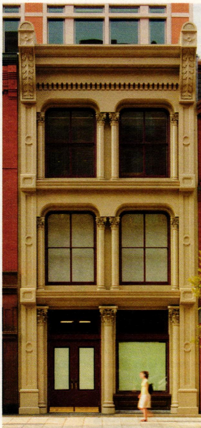
Robinson Iron cast and fabricated this new storefront façade in aluminum to match the surrounding historic neighborhood in Washington, DC.
