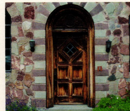
HeartWood Fine Windows & Doors made this 2 1/4-in. thick mortise-and-tenon solid-wood door of sawn white oak to replicate the original door made 100 years ago.
