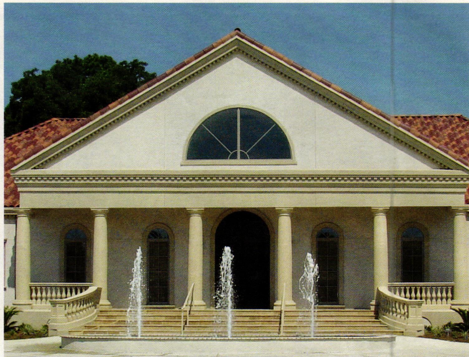
The cast-stone Tuscan columns for this building were fabricated by Melton Classics. Photo: Melton Classics
