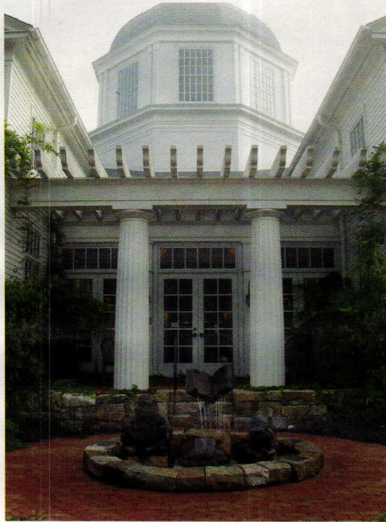
Chadsworth produced these custom fluted Greek Doric Columns with Greek Doric capitals in fiberglass for the Poland Public Library in Poland, OH. Photo: Chadsworth Columns
