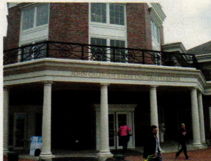
Edon Corp. supplied the fiberglass columns, cornice and spandrel panels for the John Calhoun Baker University Center at Ohio University.
