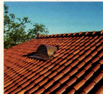
Tile Roofs supplied the natural red Spanish tile and fittings for this tile roof restoration in New Orleans, LA.
