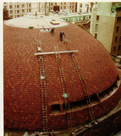
The dome of the New York City Center was originally finished in Ludowici Roof Tile in 1923; it was restored with roof tile from the same company in 2004.
