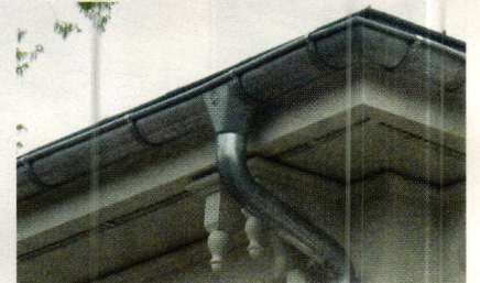
Ornametals supplied the standing-seam gray zinc (VMZINC) roofing and rainwater system for the historic antebellum Cooper House in Huntsville, AL, when it was restored by the Central Presbyterian Church.
