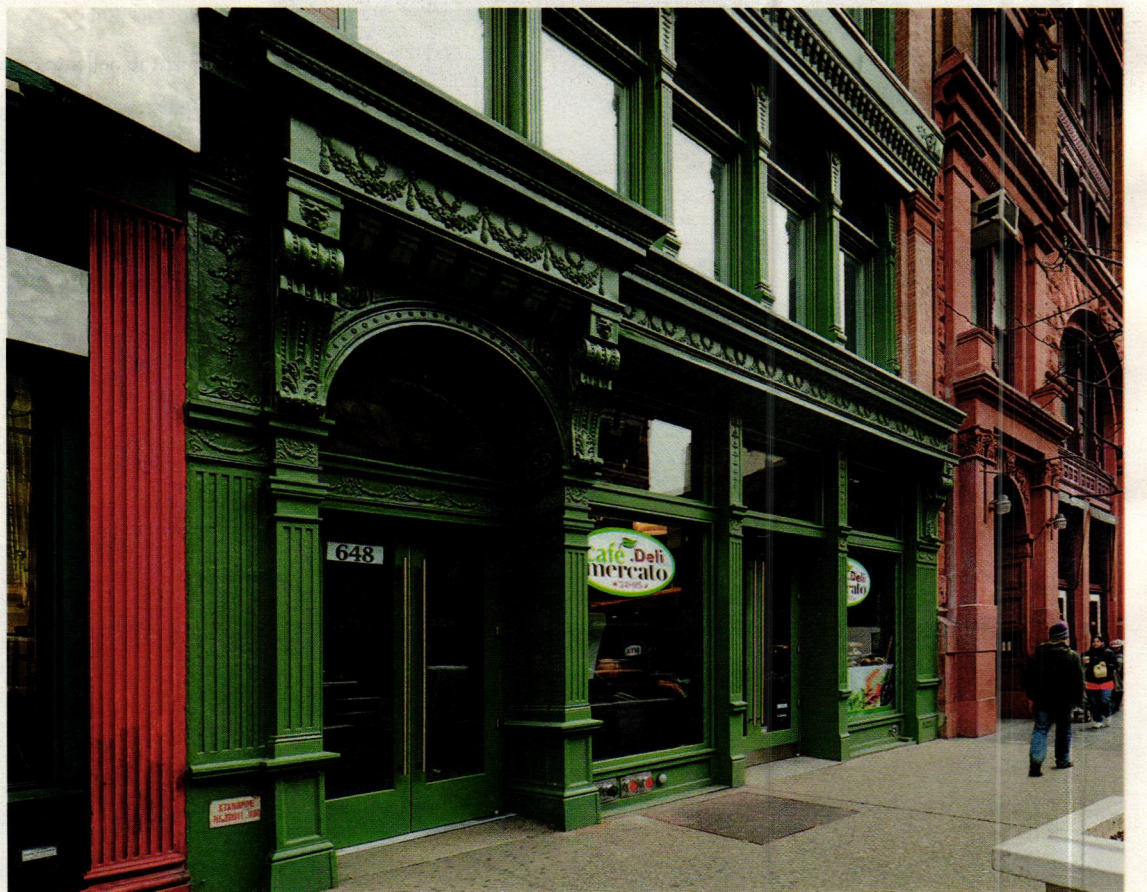
Right: The storefront has been freed of 20 th -century accretions, and an ADA-compliant ramp snuck over a basement lateral beam at the dell doorway at right. Photo: Jack Kucy
