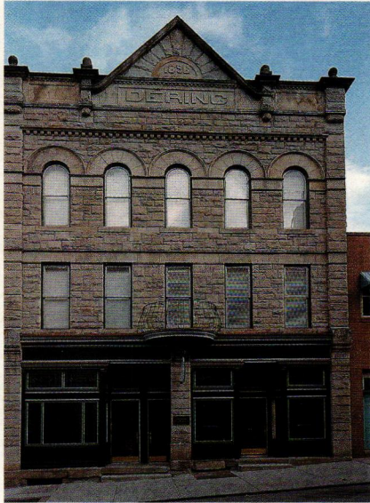
Allegheny Restoration restored and renovated the millwork, windows and entrance of the Dering Building in the historic city of Morganstown, WV.
