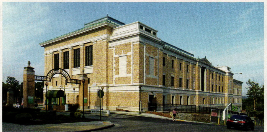
TOP: North Hall extends the axis and continues the architectural vocabulary established by Stanford White's Hall of Fame for Great Americans, completed in 1900. It and White's Gould Memorial Library are New York City landmarks that are on the National Register of Historic Places.
