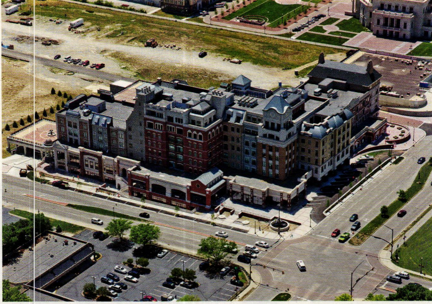
ABOVE: A vision of Mayor Jim Brainaird, the Carmel City Center complex in Carmel, IN, was developed by Pedcor Design Group to satisfy the city's need for a pedestrian-oriented downtown. All photos: courtesy of Pedcor Design Group
