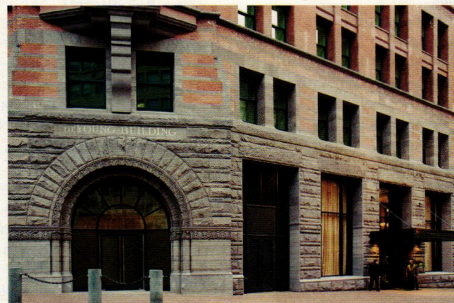
Kopelov Cut Stone quarried and fabricated the brownstone for the renovation of the old Chronicle Building, San Francisco, CA.
