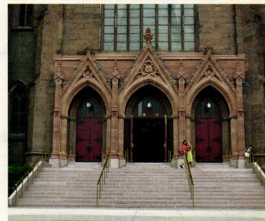
Old World Stone provided the cut and carved St. Bee's sandstone and granite steps (shown here) for the entry portico of the Cathedral of the Immaculate Conception in Albany, NY.
