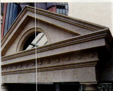
This custom cast-stone pedimented entrance to a shopping mall was fabricated by Haddonstone.
