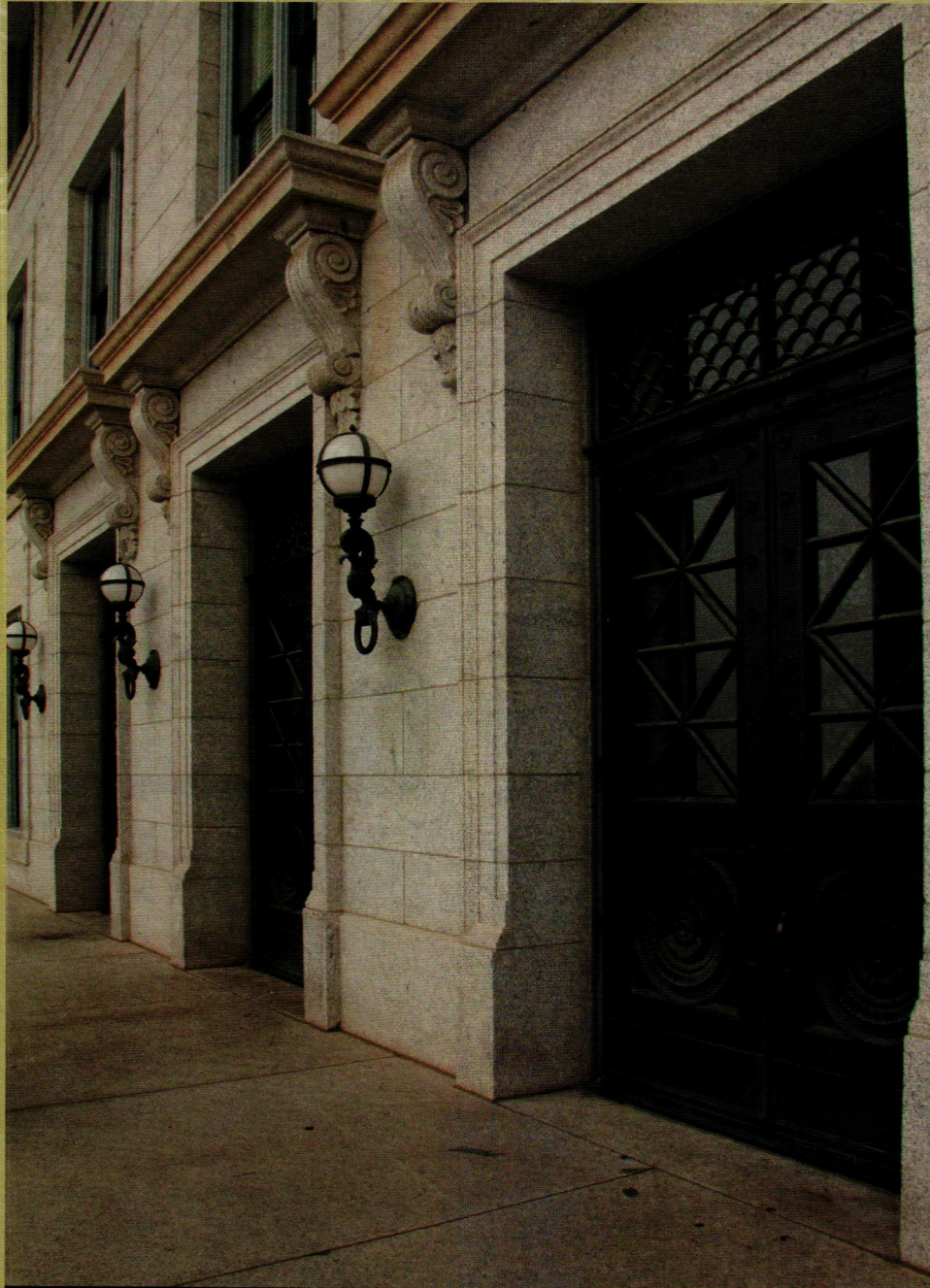
STATE CAPITOL, SALT LAKE CITY, UTAH / HISTORICAL BRONZE DOOR RESTORATION
