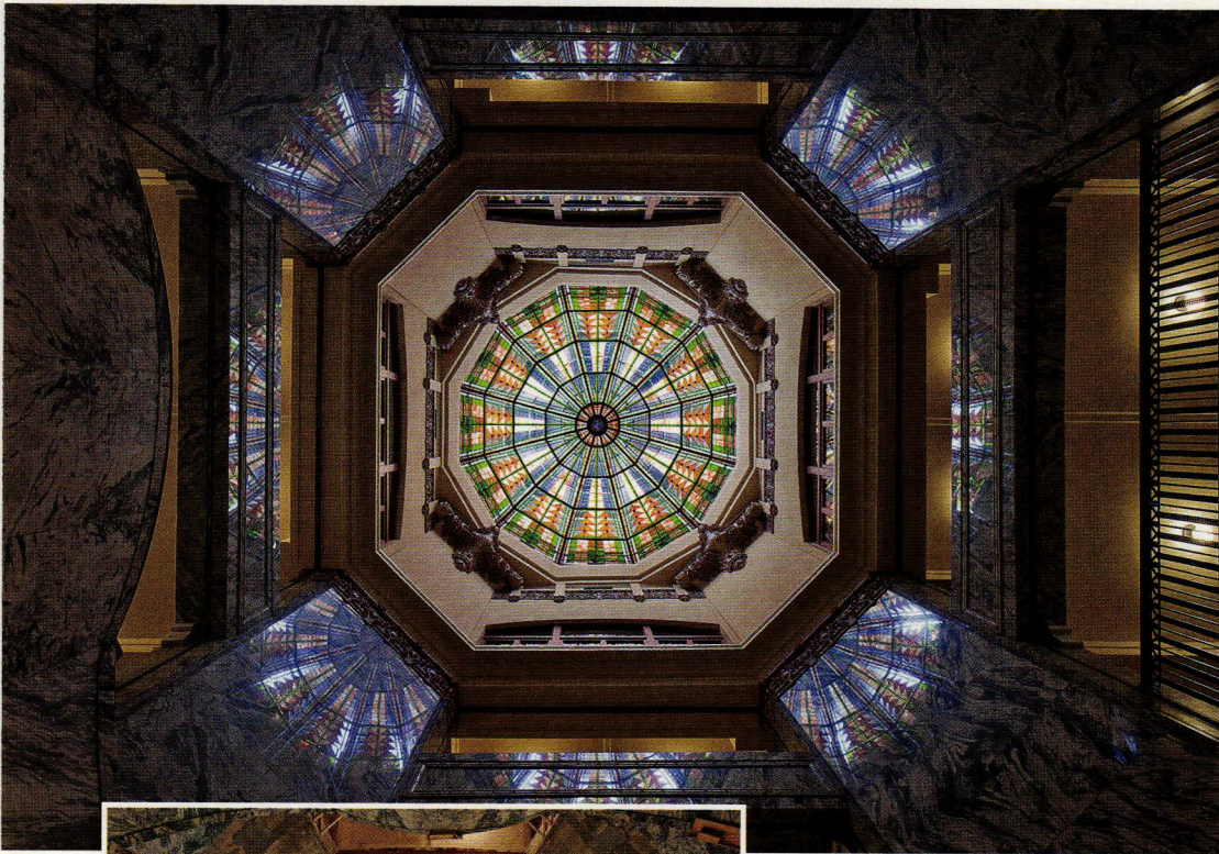
ABOVE: The design of the new art-glass dome in the rotunda is interpretive. No documentation of the original 80-ft. dia. dome was found so the architects visited two other Texas courthouses to guide them in the design.
