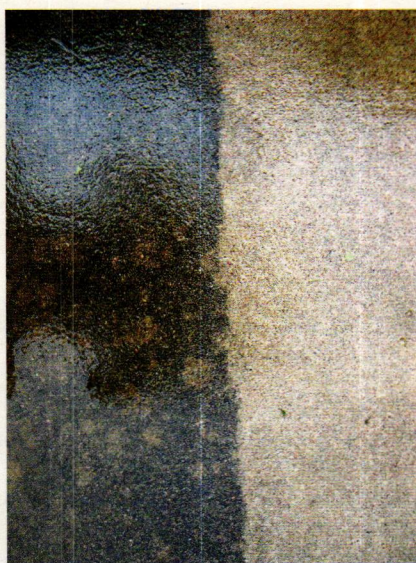
Prosoco's EK2010 was used to repair this concrete patio.
