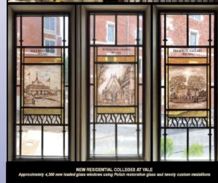
NEW RESIDENTIAL COLLEGES AT YALE Approximately 4,300 new leaded glass windows using Polish restoration glass and heavy custom muntins
