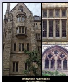
BRANFORD / BAYBROOK Over 7,000 windows
