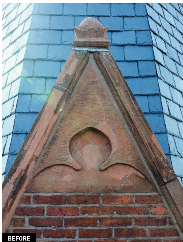
ABOVE One of the more challenging aspects of this project was trying to recreate the heavily damaged finials on the main tower. They had been patched and re-carved so many times that they no longer resembled anything like the original highly ornamental finials. The restoration team only had one historic low-resolution image to help guide the replacement.
