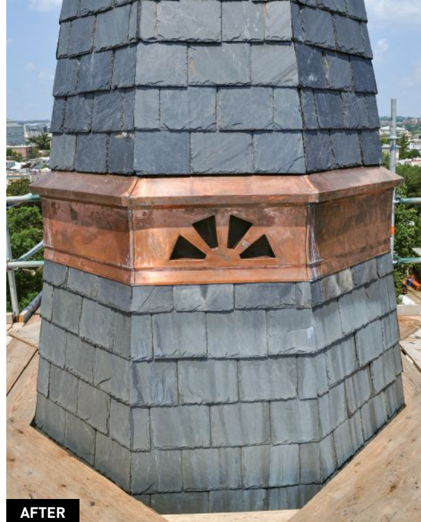
ABOVE The main tower of Mark’s Episcopal Church in Washington, D.C., had four turrets that were extensively repaired and restored by the Aeon Preservation team. This entailed rebuilding wooden framing, new copper roofing and cladding, fabrication of new decorative stones, and rebuilding large sections of masonry.
