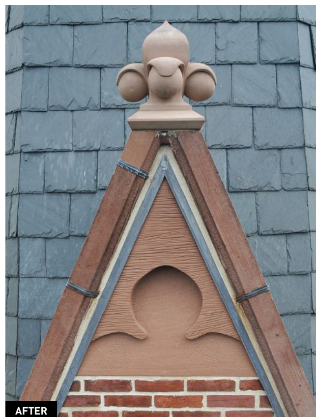
ABOVE One of the more challenging aspects of this project was trying to recreate the heavily damaged finials on the main tower. They had been patched and re-carved so many times that they no longer resembled anything like the original highly ornamental finials. The restoration team only had one historic low-resolution image to help guide the replacement.
