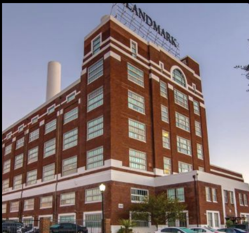
Landmark Lofts - New Braunfels, TX
