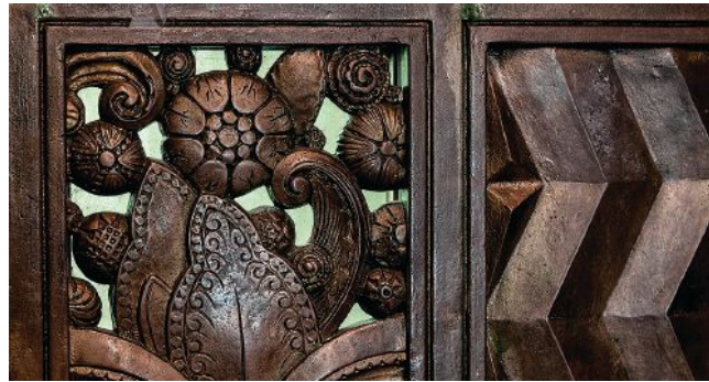
ABOVE Original bronze work (left) and light fixtures were carefully restored.
